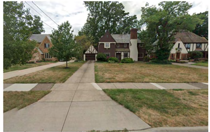
From Street - West
