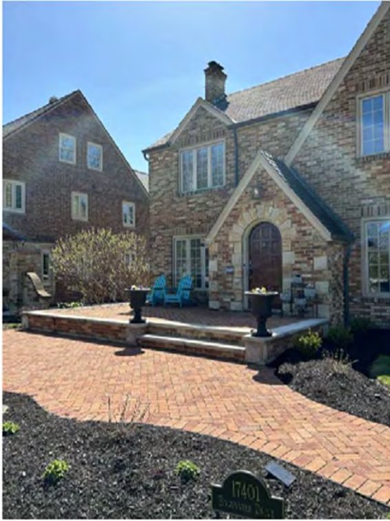
Existing Patio - From West
