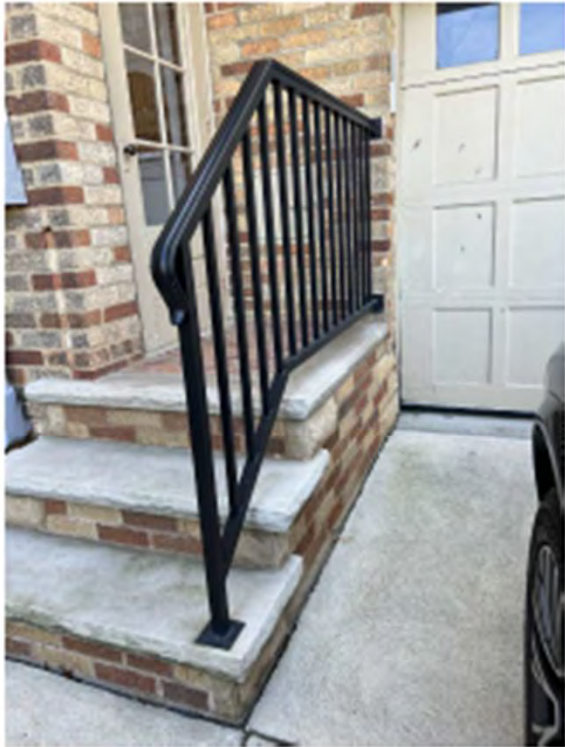
Existing Iron Railing - Custom (match)
