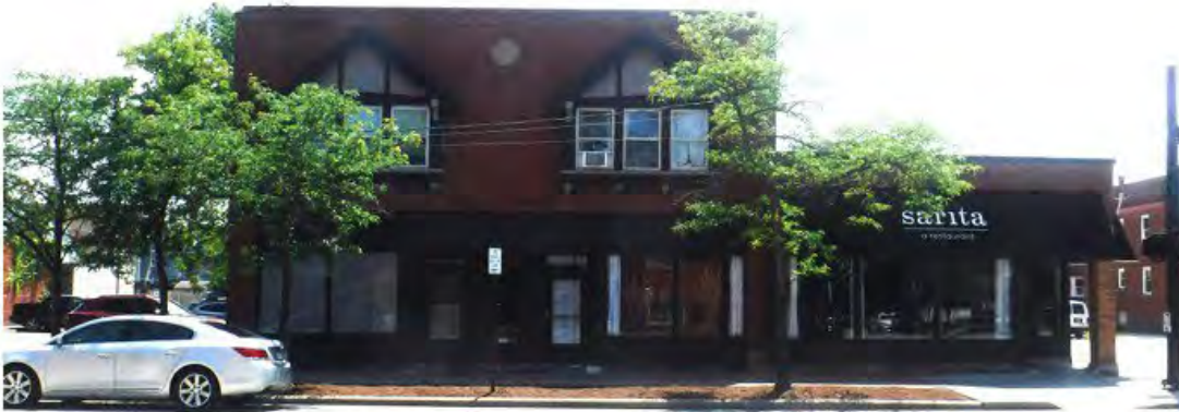
EXISTING CONDITIONS PHOTO VIEWING SOUTH N.T.S.
