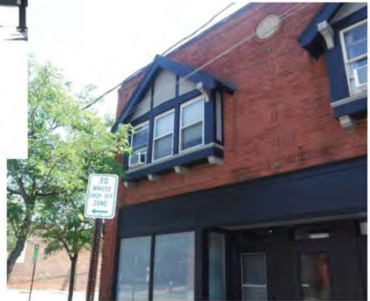
EXISTING CONDITIONS PHOTO VIEWING SOUTHEAST N.T.S.
