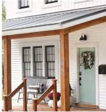
Wood Post and Metal Roof
