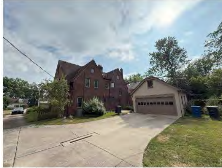
NORTH FACE OF EXISTING HOUSE
