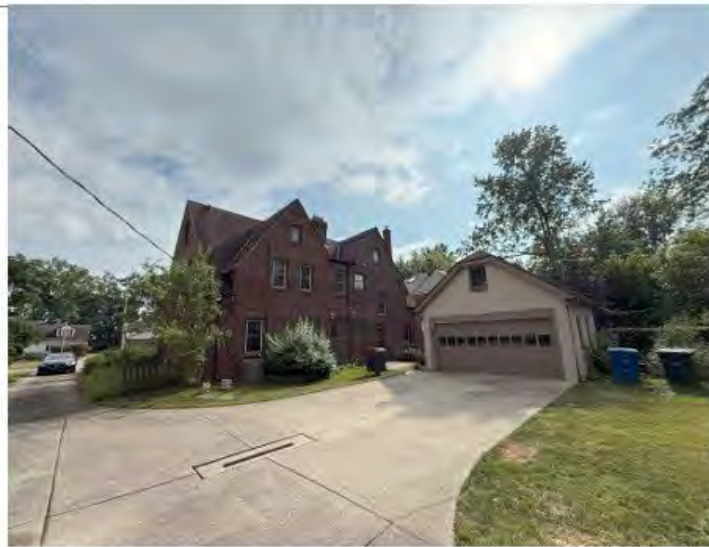
NORTH FACE OF EXISTING HOUSE
