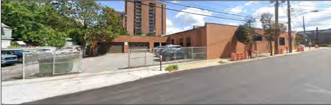
PHOTO OF EXISTING WEST ELEVATION
