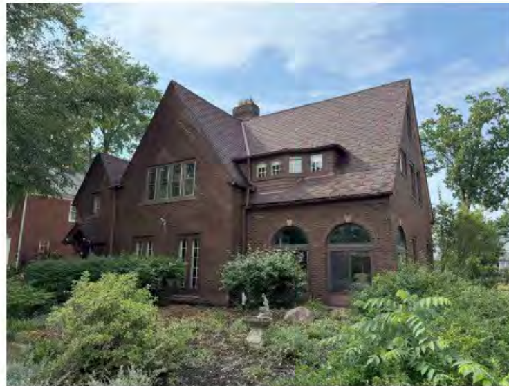
SOUTH FACE OF EXISTING HOUSE
