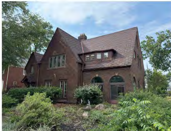
SOUTH FACE OF EXISTING HOUSE
