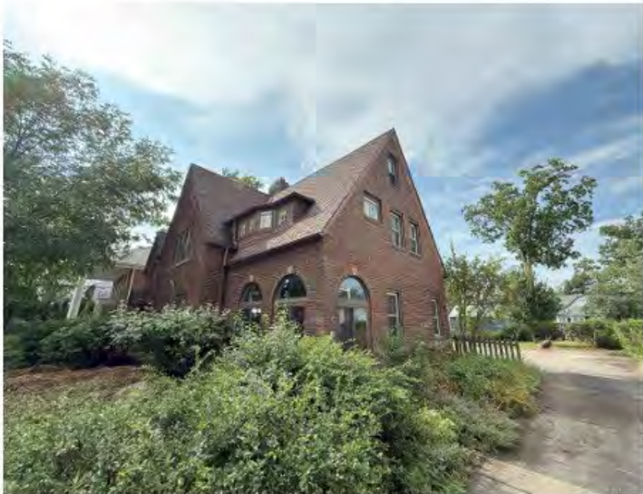
EXISTING HOUSE DORMER
