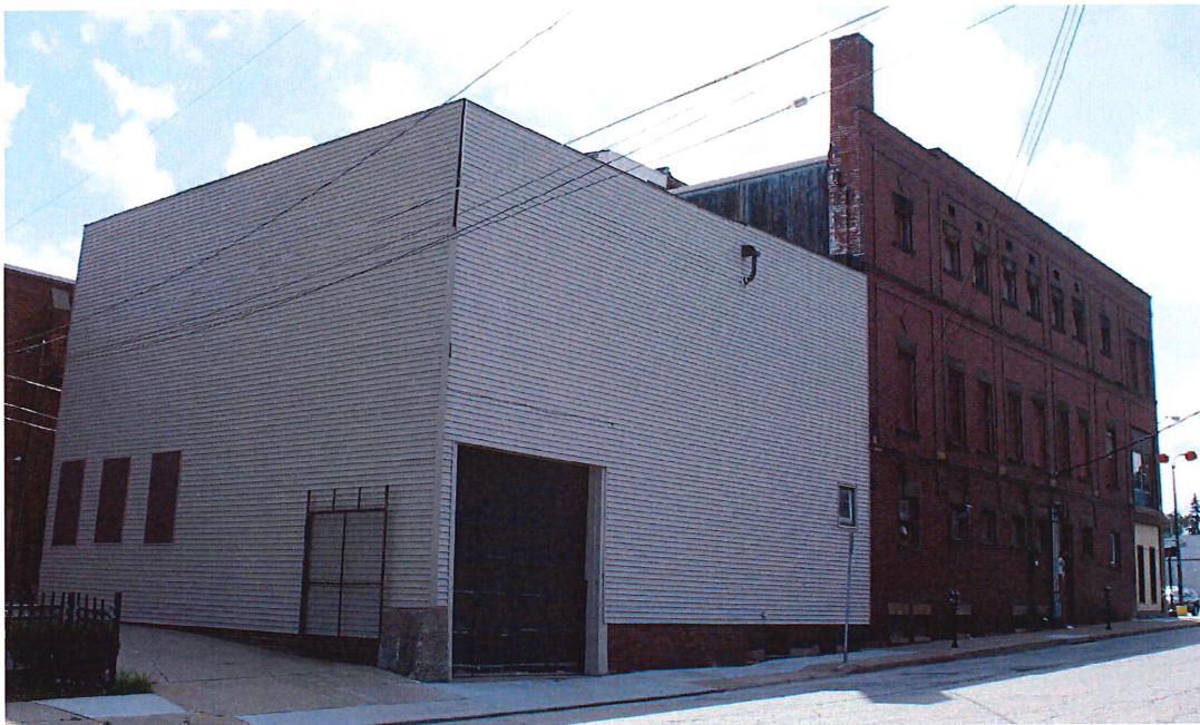
Photo 3: North and West Elevations, 2017.
