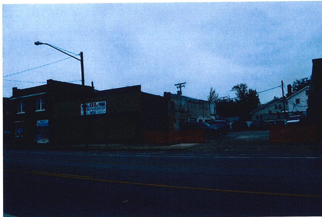
Side and Front View of Building at 13415 Madison Avenue, Lakewood
