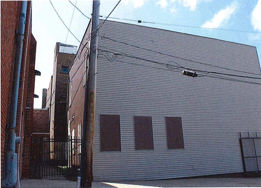
Photo 4: North and East Elevations, 2017.
