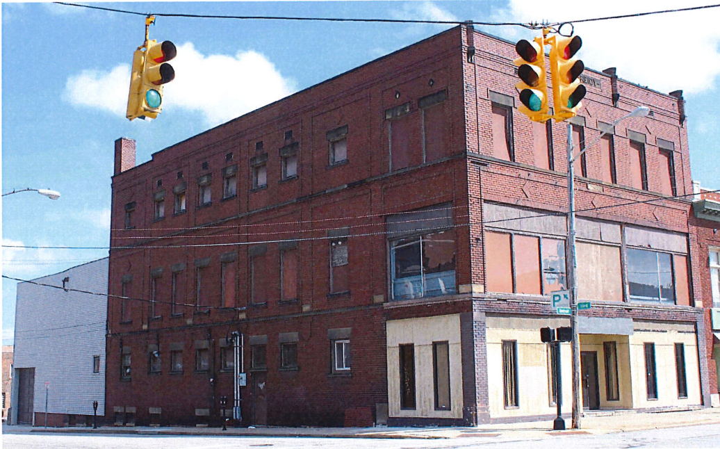
Photo 2: South and West Elevations, 2017.
