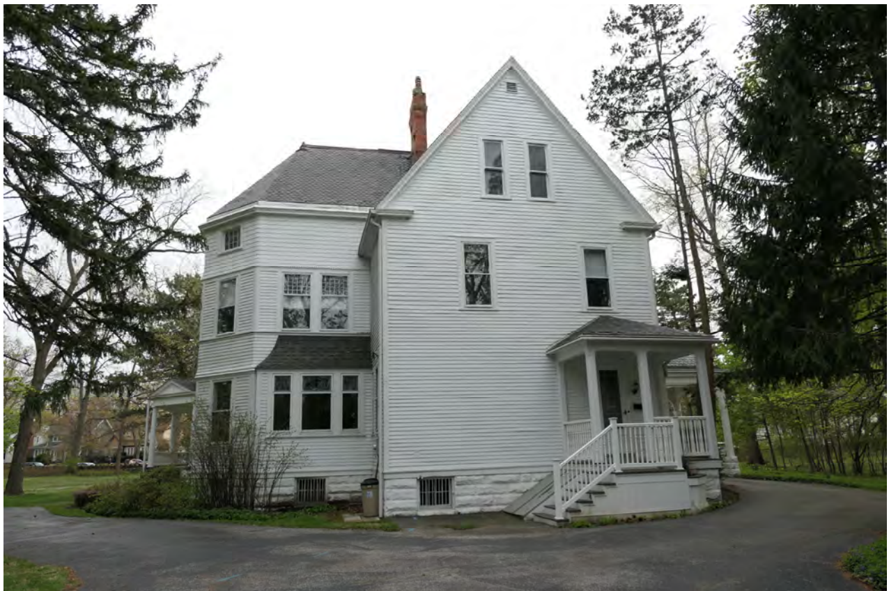
4. North elevation, camera facing south
