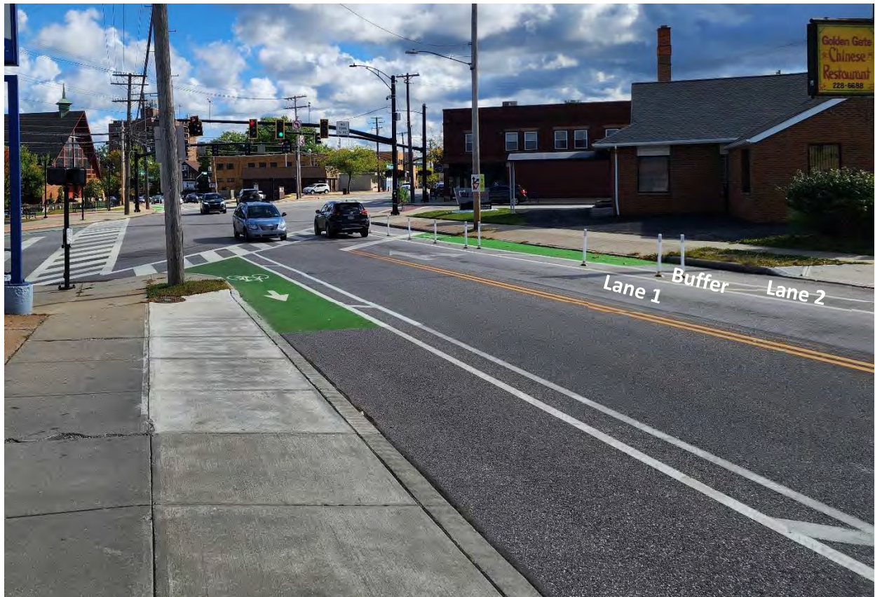
Figure 5 – Hilliard Rd Northeast Approach
