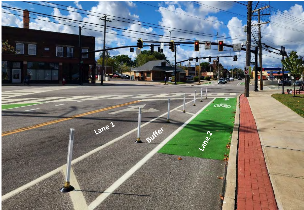
Figure 6 – Hilliard Rd Southwest Approach
