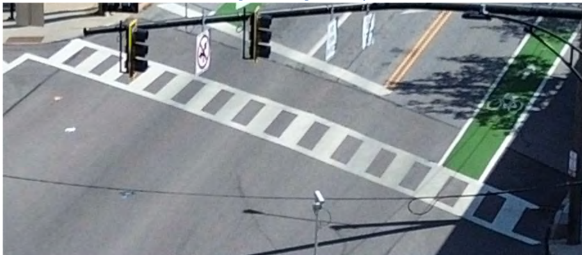
Figure 19 – High Visibility Crosswalk
