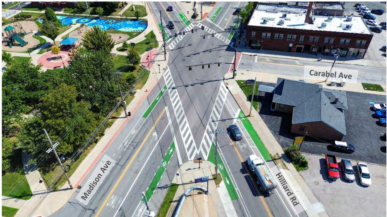
Figure 2 – Madison Ave & Hilliard Rd/Carabel Ave Aerial View
