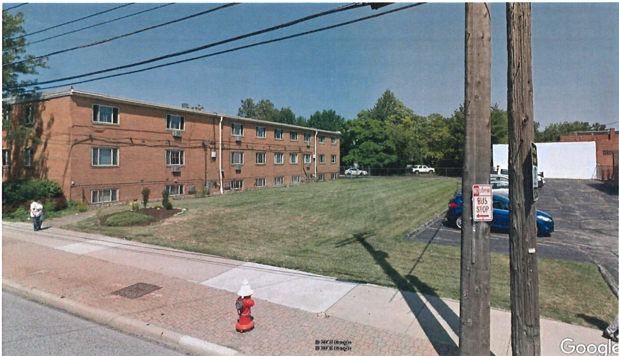
STREET VIEW FACING NORTHWEST
