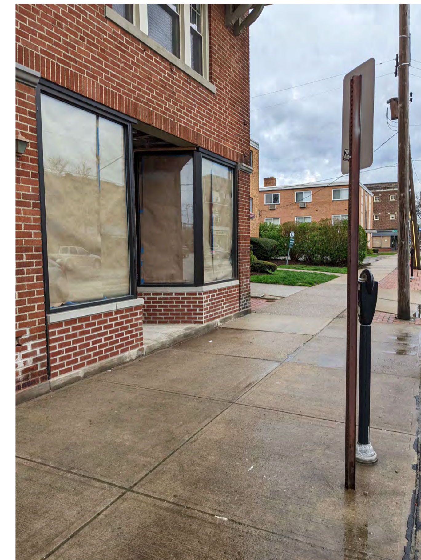
Existing Photo Looking West
