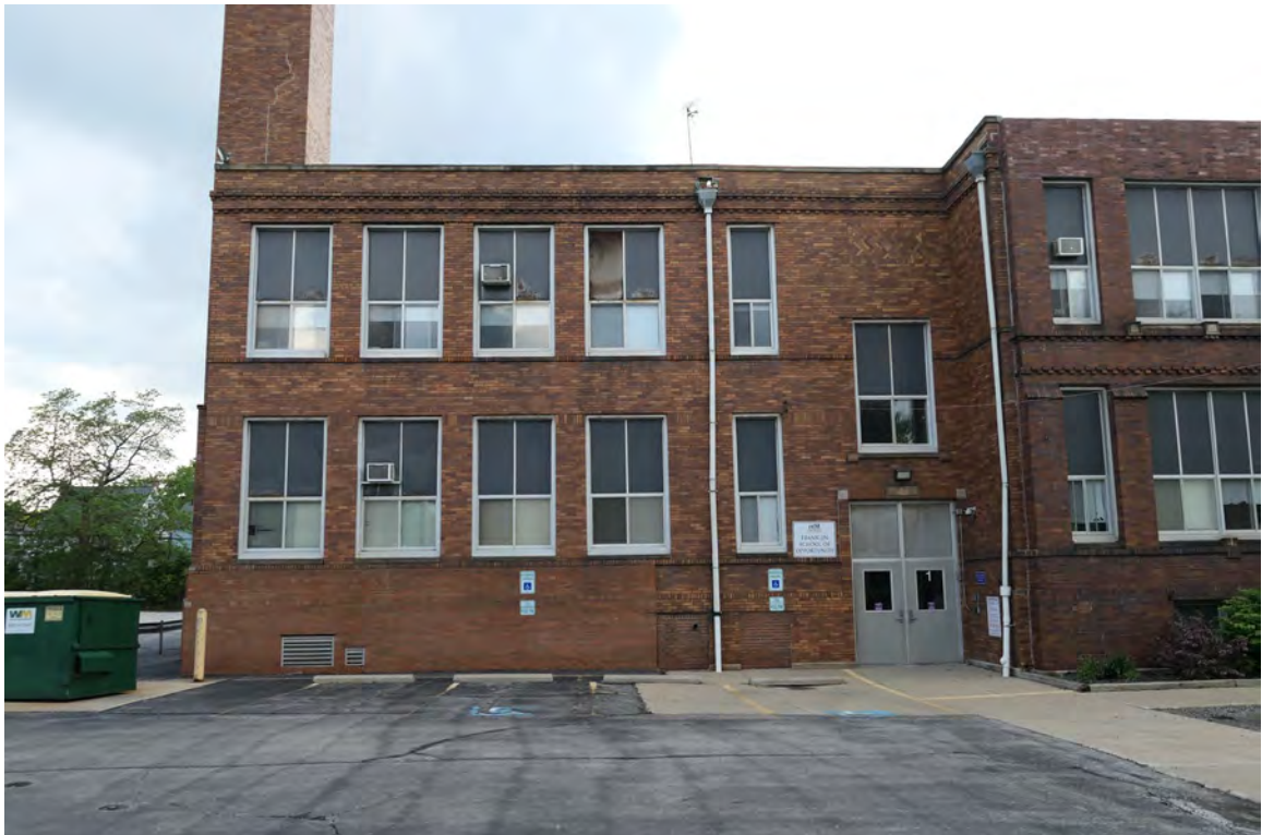
8. East elevation, 1920 addition, camera facing west
