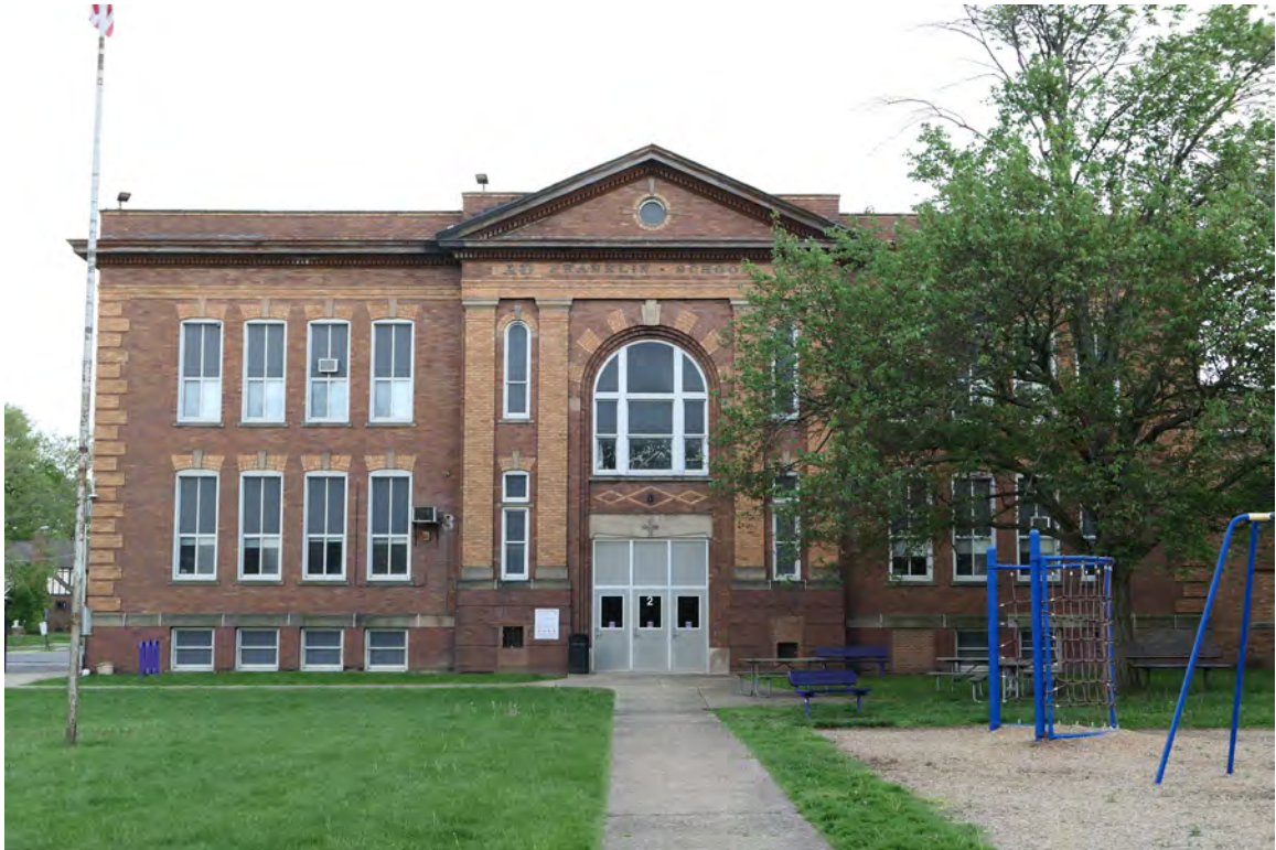
3. North façade, original 1907 building, camera facing south
