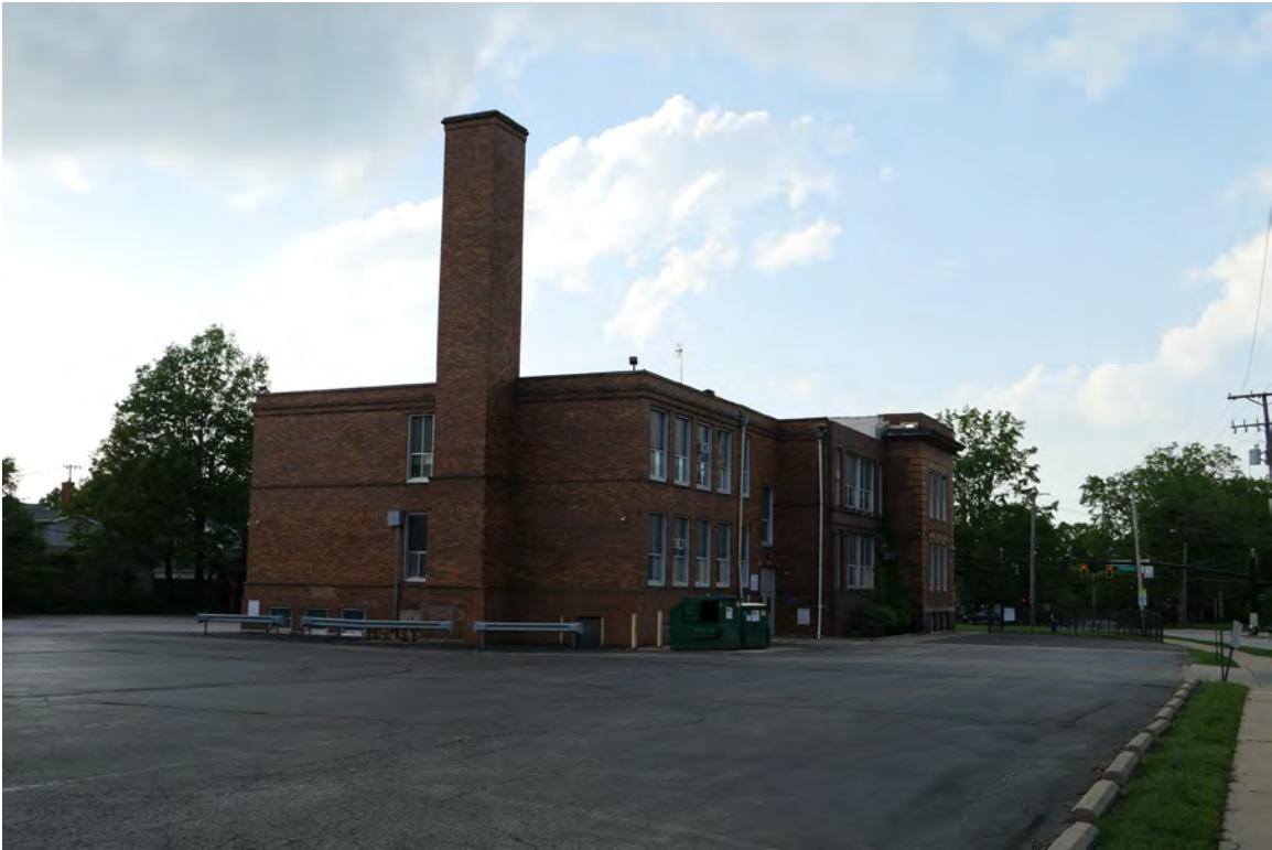
9. Southeast oblique, rear elevation and site, camera facing northwest
