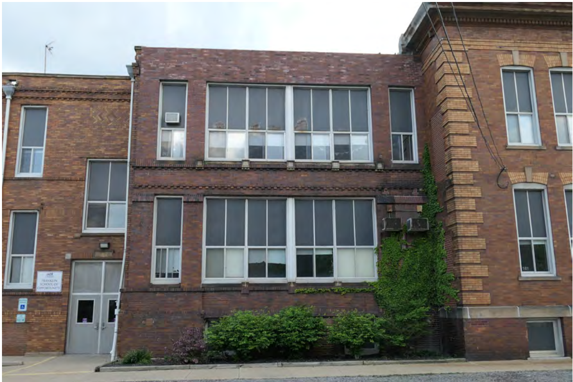
7. East elevation, 1915 addition, camera facing west
