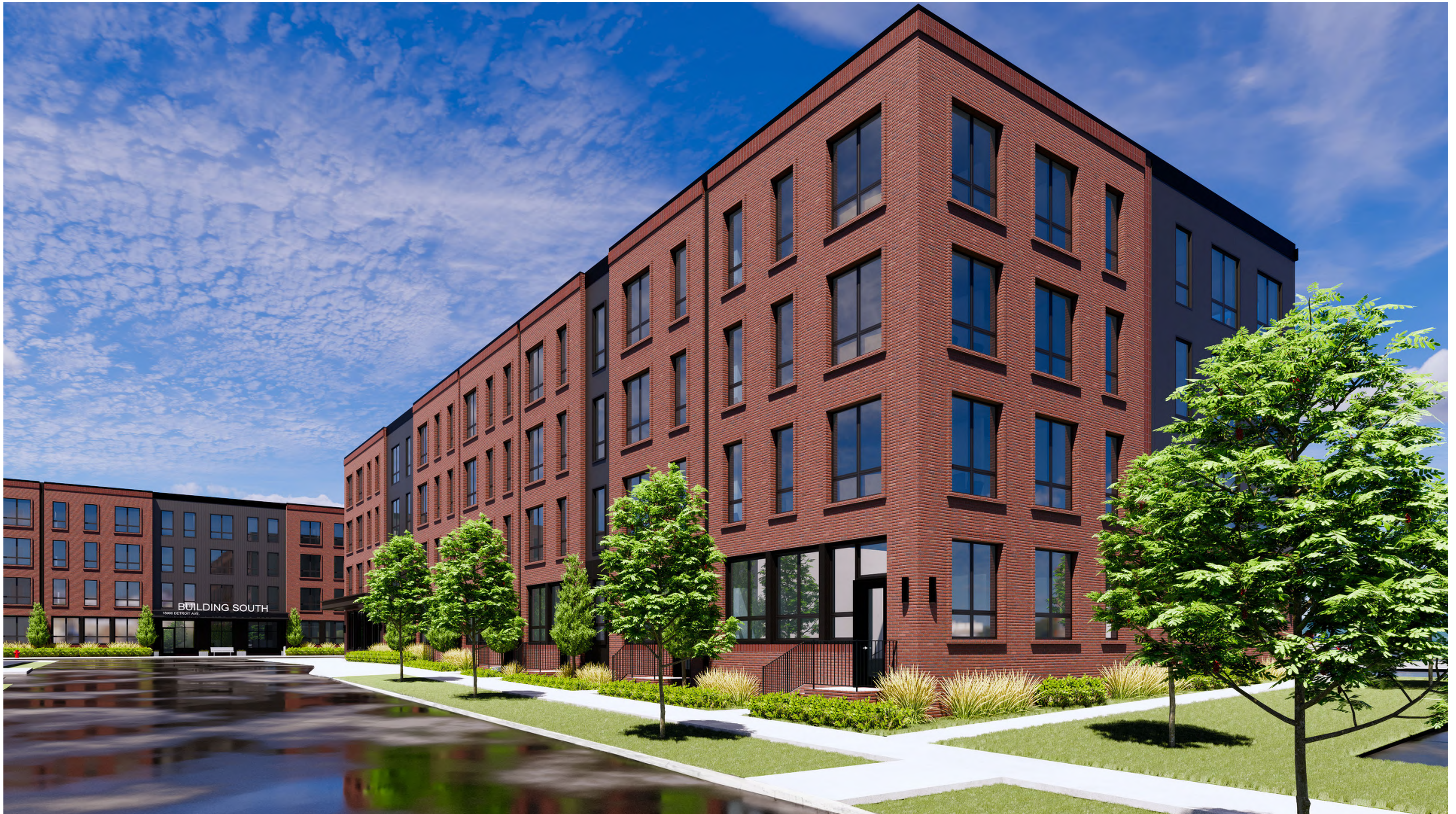
BUILDING NORTH - VIEW LOOKING SOUTH ON BROCKLEY AVENUE
