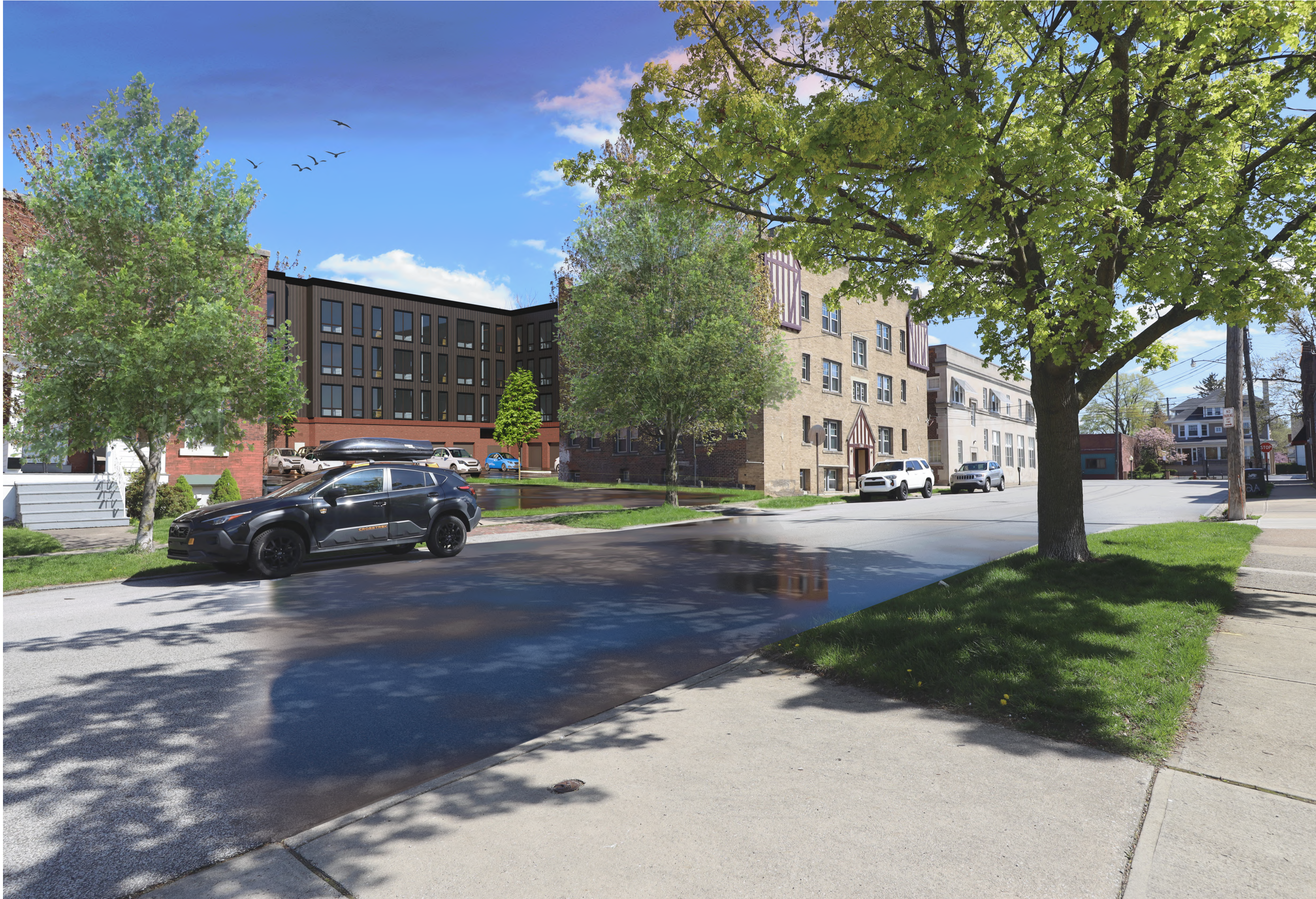
6. BUILDING NORTH - CRANFORD AVENUE LOOKING SOUTH
