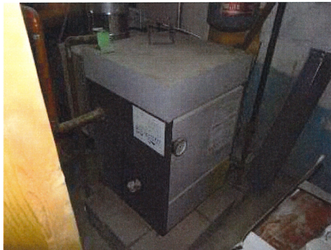
This type of system has an average typical lifespan of 25-30 years.
