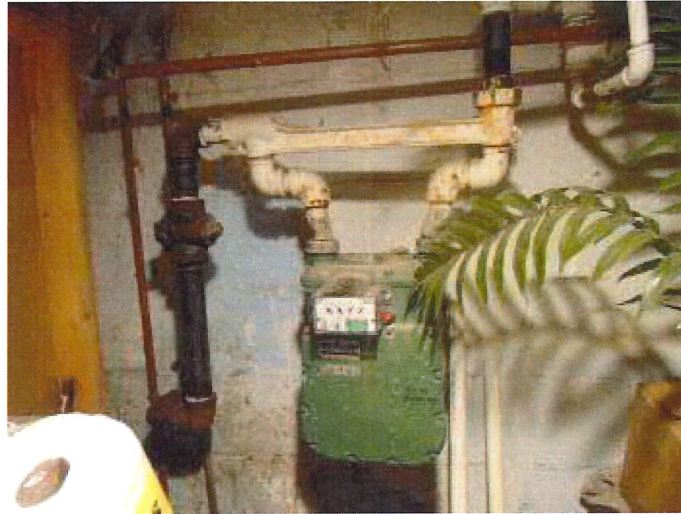
The gas meter was installed in the basement.
