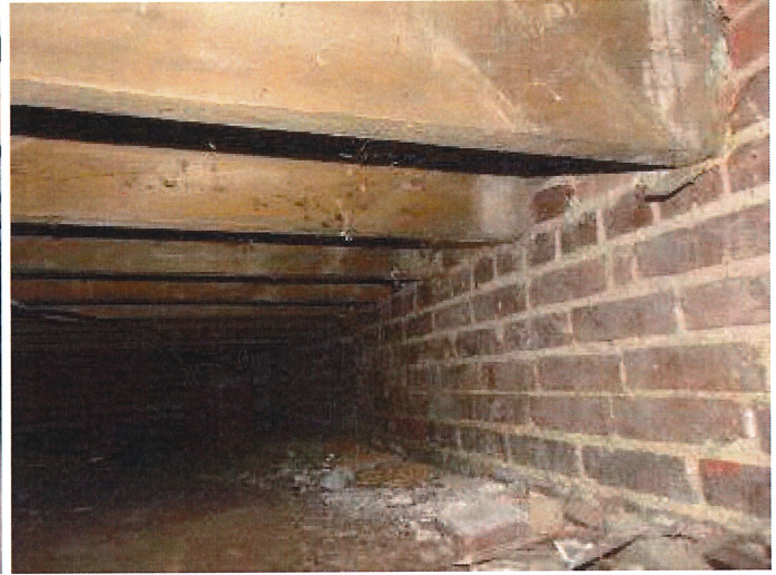
FYI picture of the crawlspace
