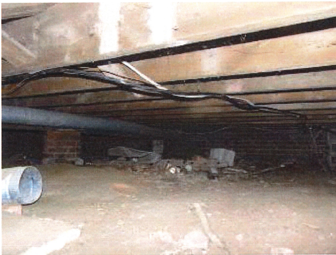
FYI picture of the crawlspace
