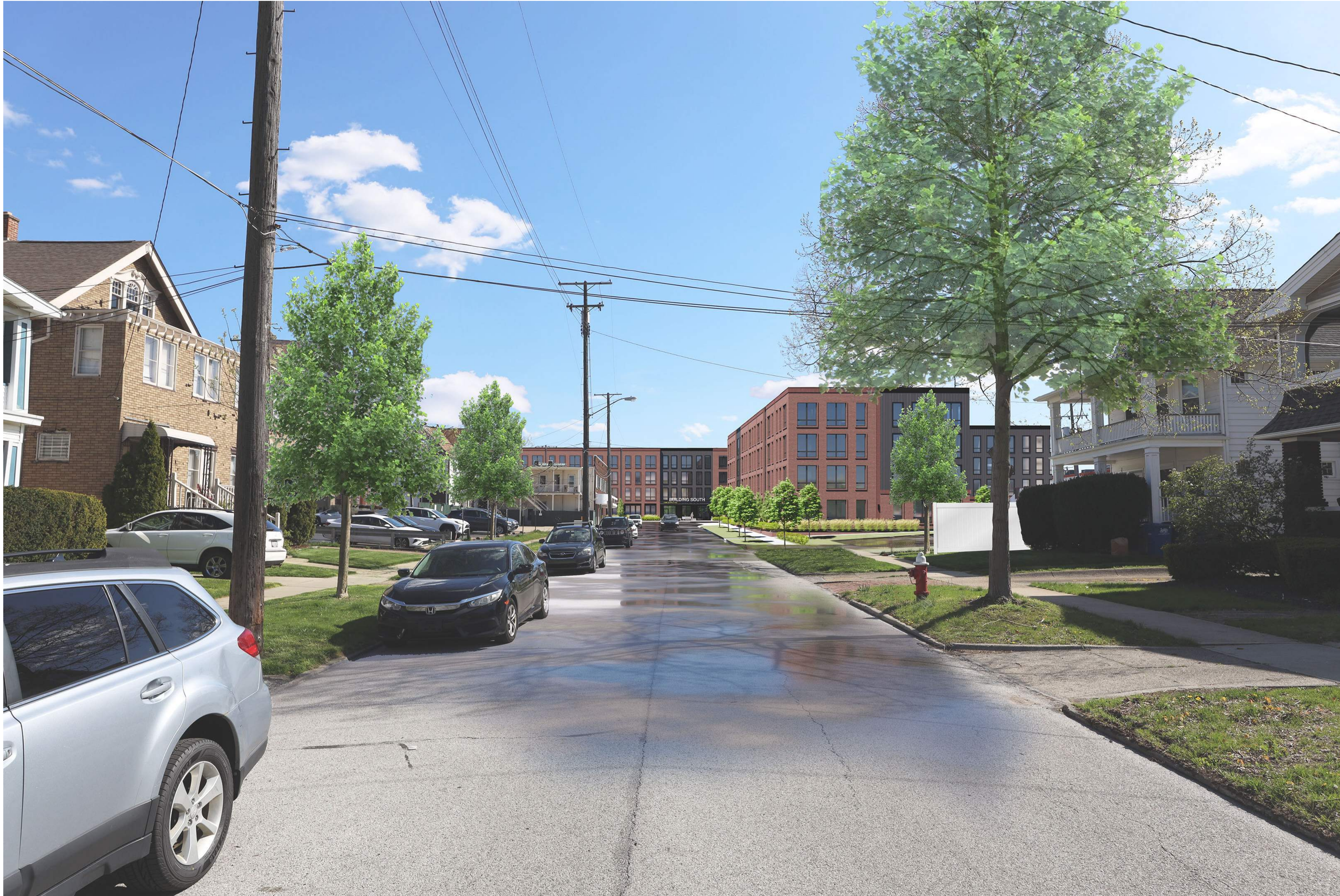
3. BUILDING NORTH & SOUTH - BROCKLEY AVENUE LOOKING SOUTH
