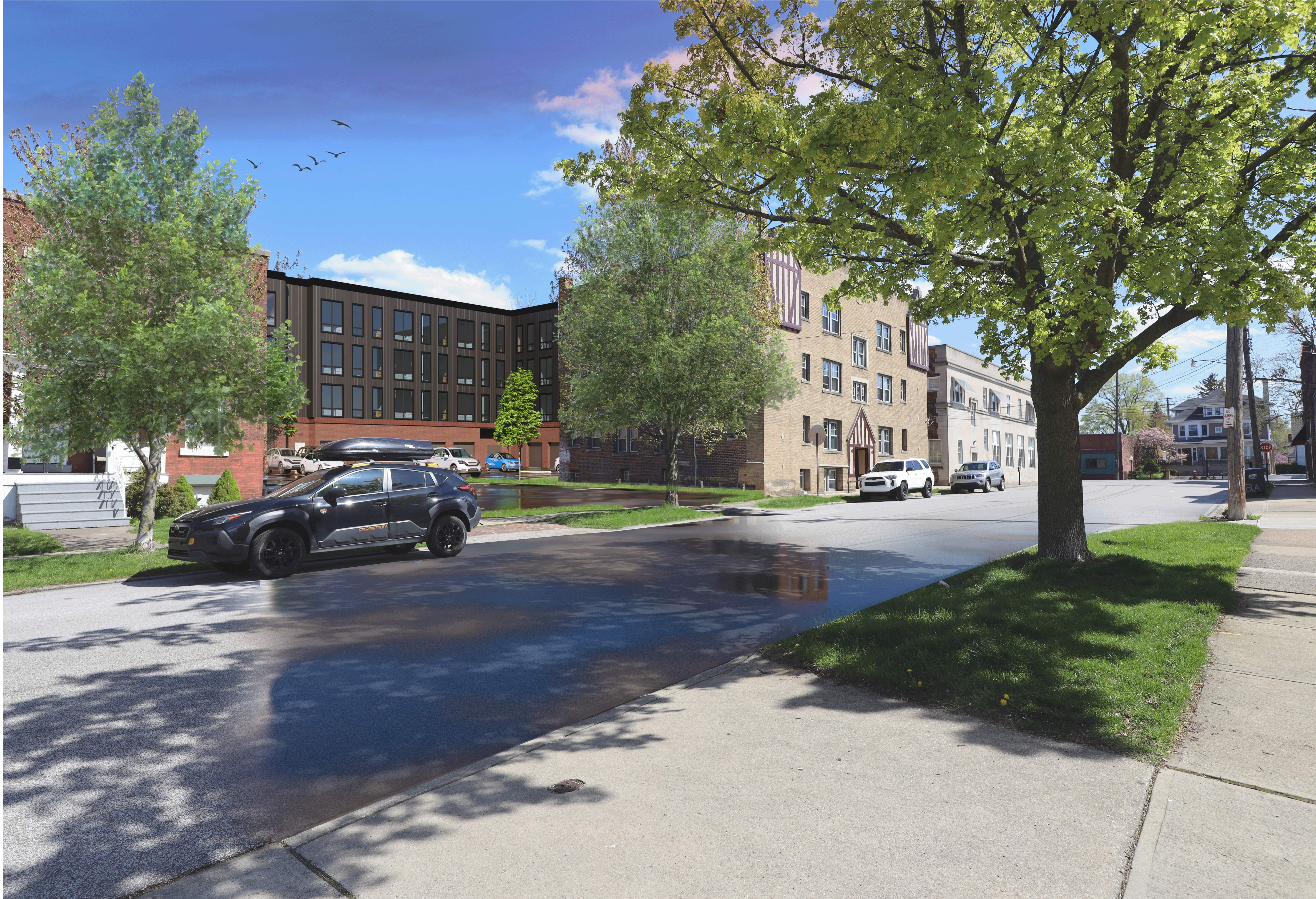
6. BUILDING NORTH - CRANFORD AVENUE LOOKING SOUTH
