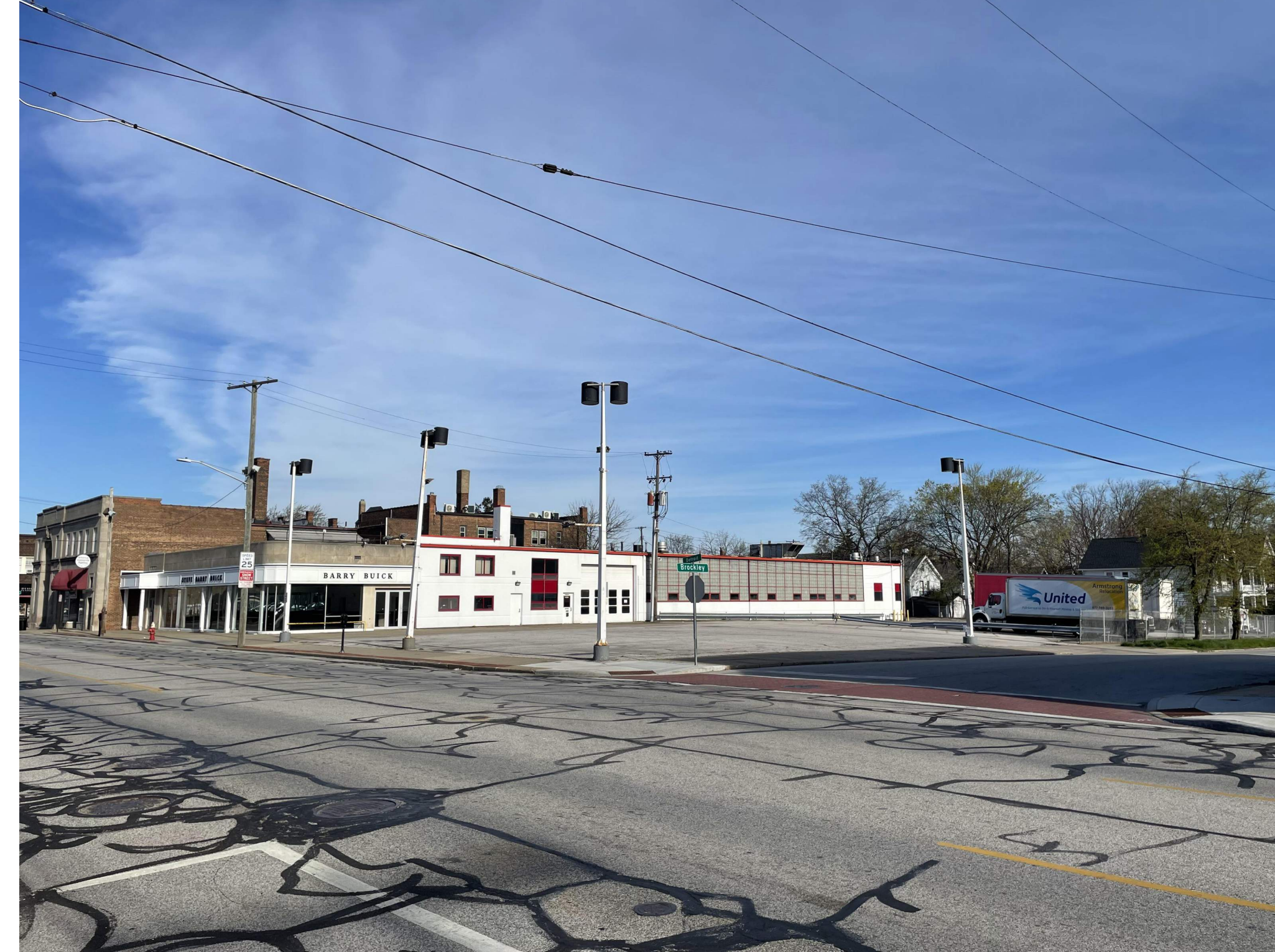
2. Brockley Avenue & Detroit Avenue Intersection
