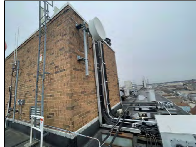
Western Penthouse Wall
