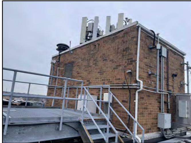
Southern Penthouse Wall
