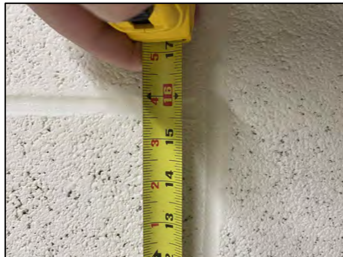
CMU Block Length (Bearing Wall)
