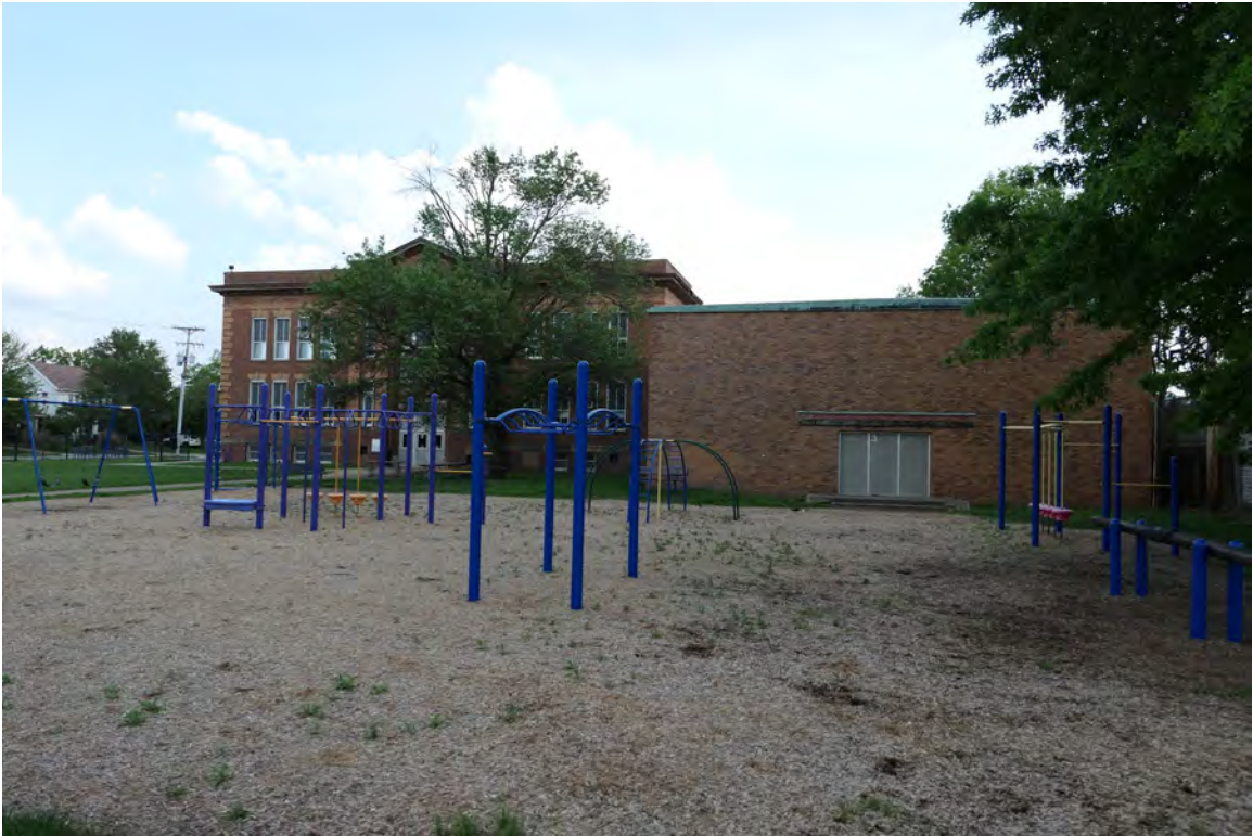
11. North elevation, modern addition and playground, camera facing south
