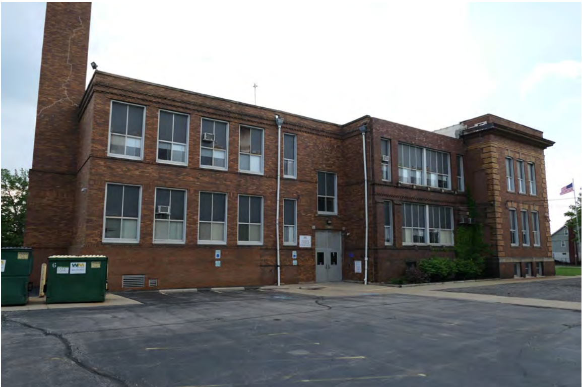
6. East elevation, with 1915 and 1920 additions, camera facing northwest
