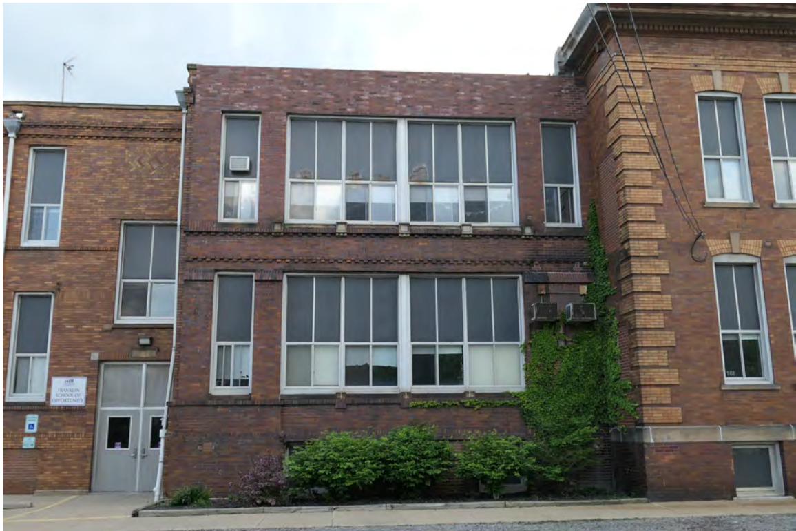
7. East elevation, 1915 addition, camera facing west
