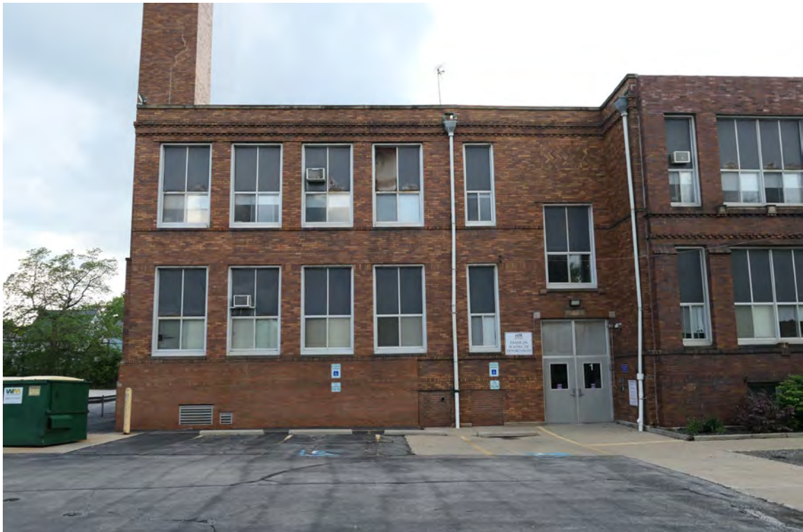
8. East elevation, 1920 addition, camera facing west
