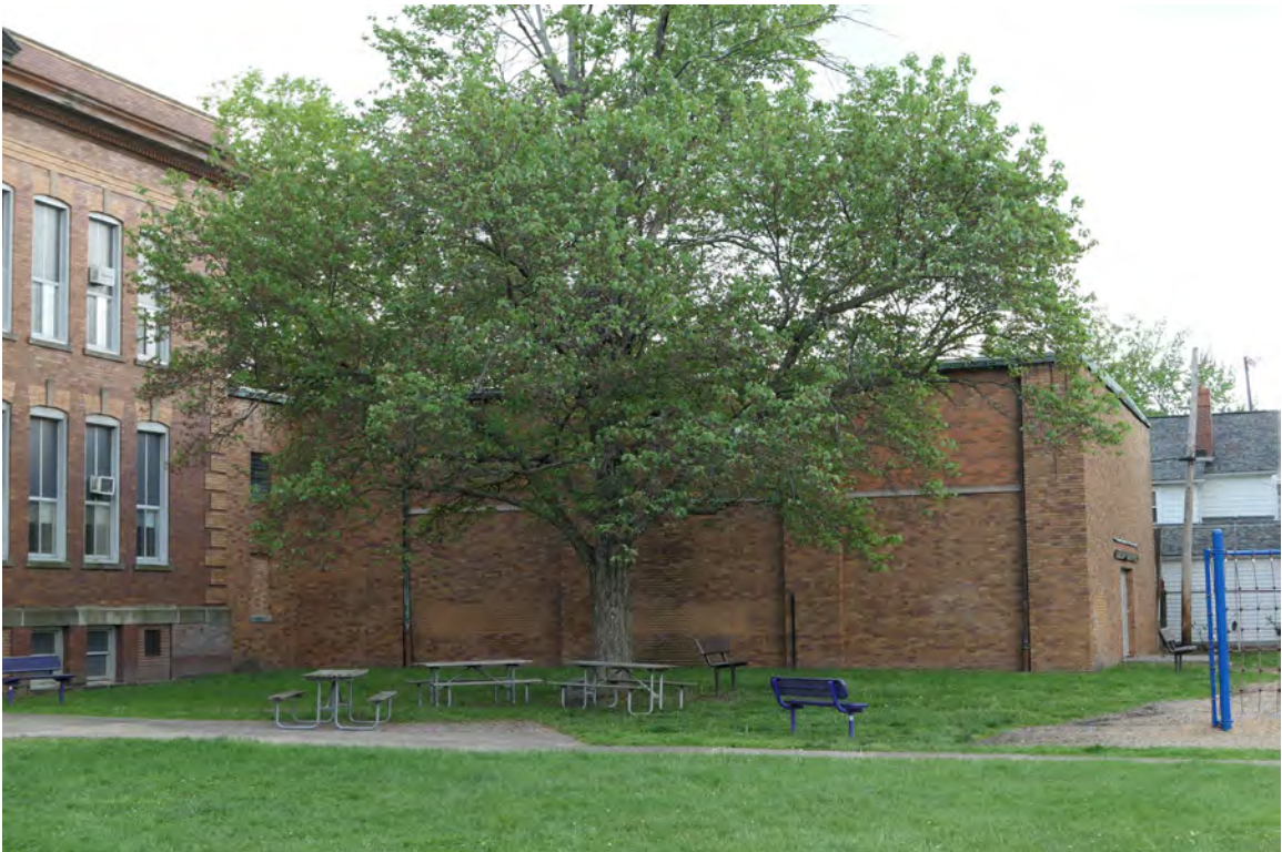
10. East elevation, modern addition to northwest, camera facing west
