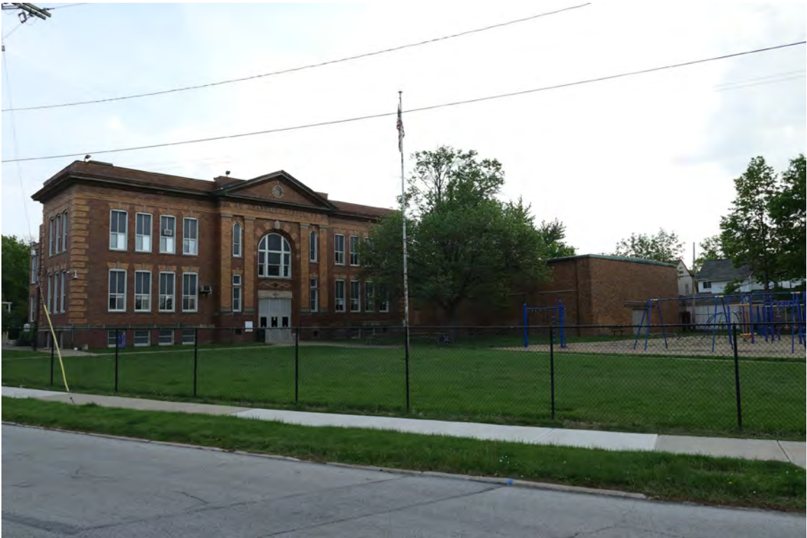
1. Northeast oblique, primary elevations and site, camera facing southwest
