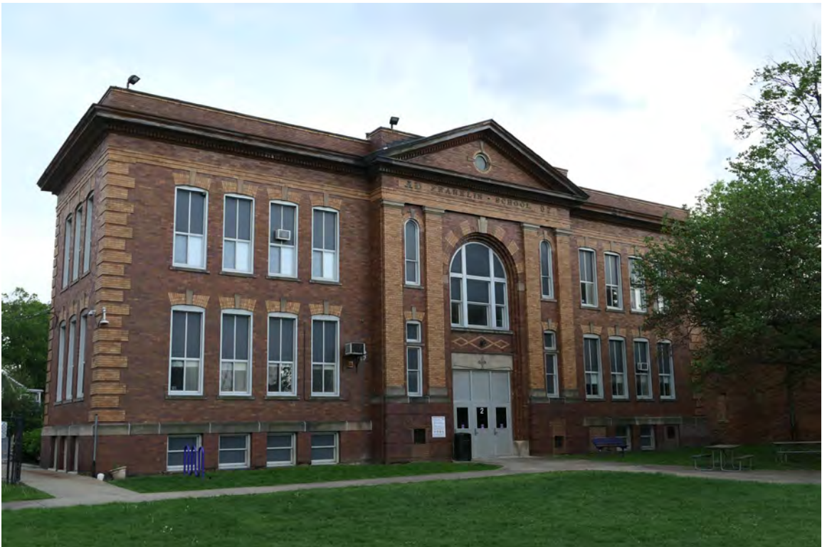
2. Northeast oblique, primary north façade, camera facing southwest
