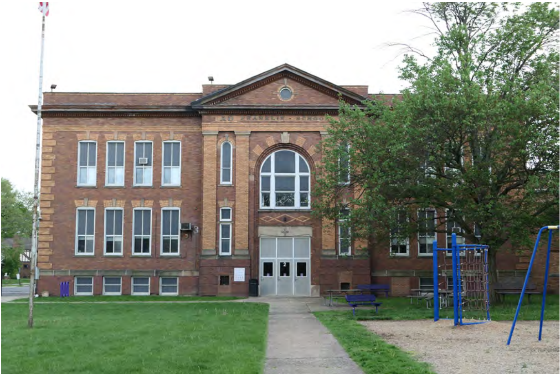
3. North façade, original 1907 building, camera facing south
