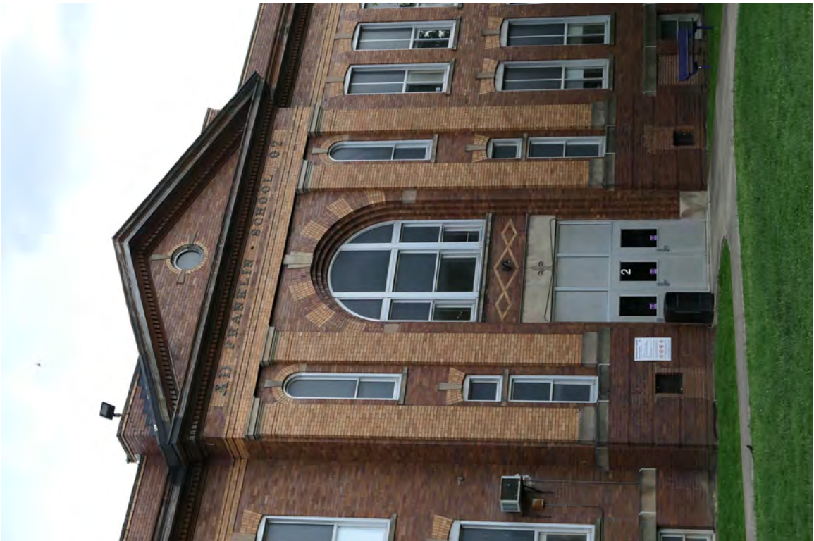
4. North façade, original 1907 building, central entry bay, camera facing southwest
