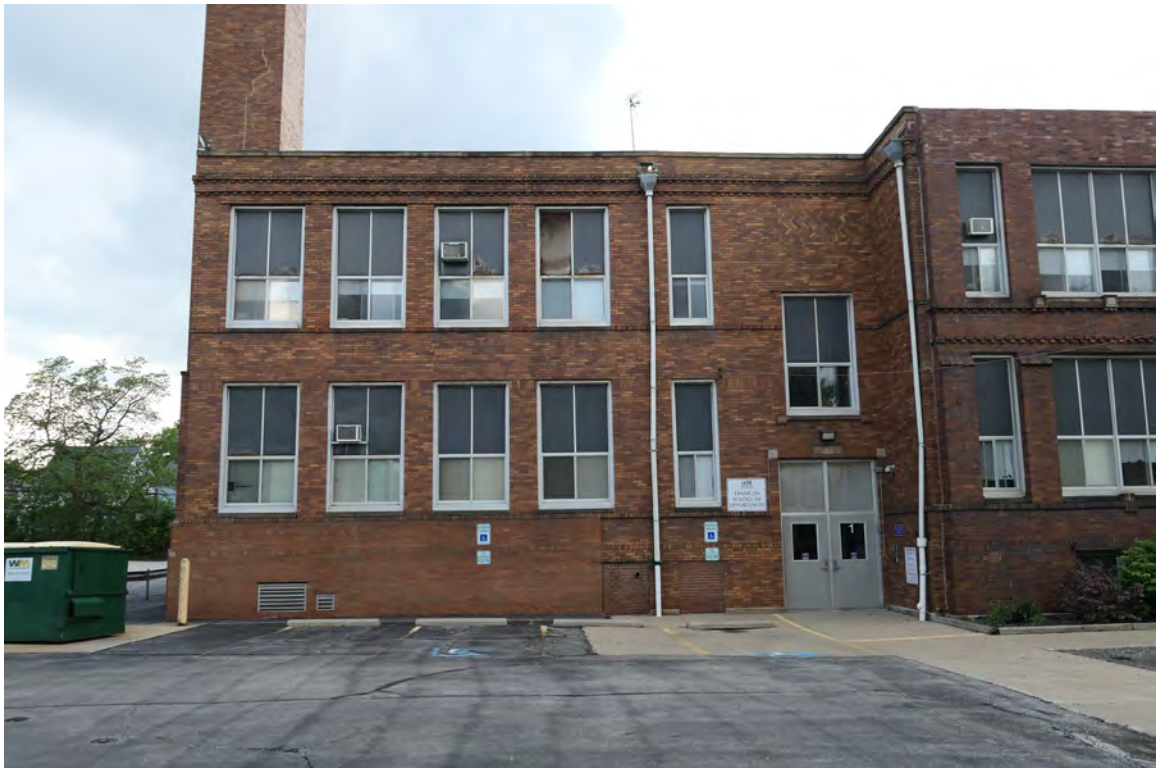
8. East elevation, 1920 addition, camera facing west
