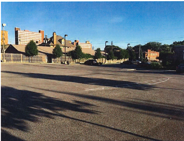
Parking lot looking Northeast
