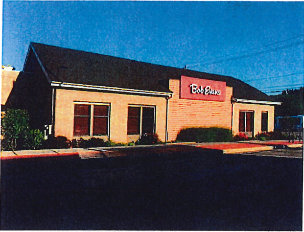
East side of building
