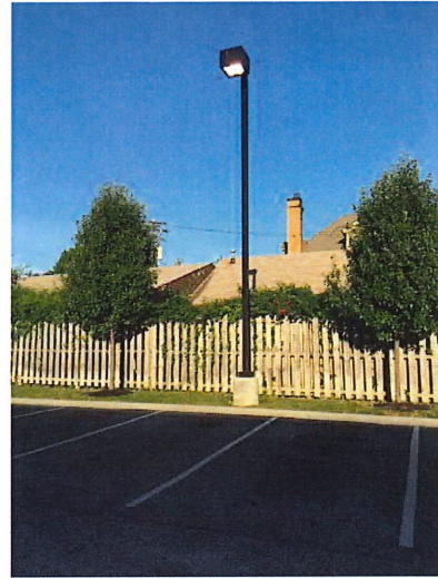
Parking lot light pole
