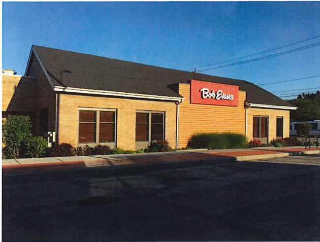
East side of building
