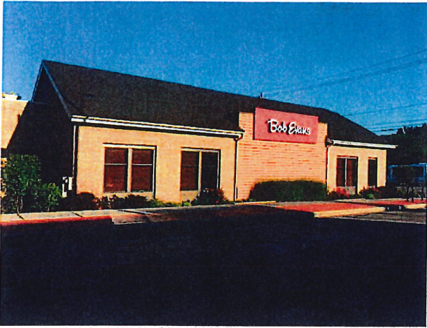
East side of building
