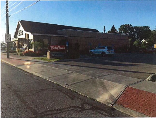
West side of building
