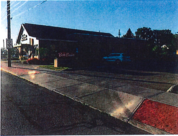
West side of building
