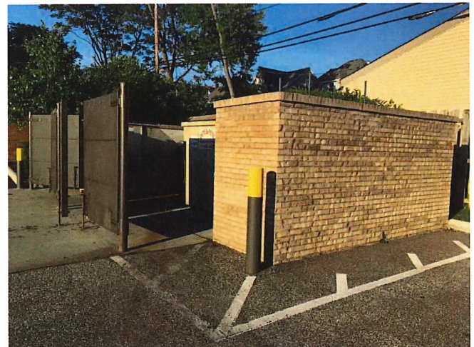
Dumpster enclosure at southwest of parking lot
