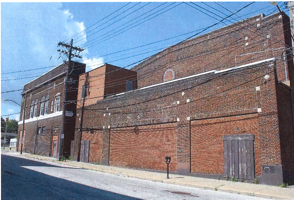
Photo 4: East elevation of theater block and gated courtyard (c.d. SW).
