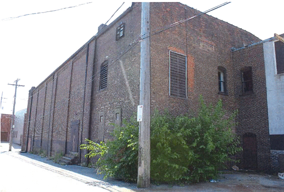
Photo 6: Northwest elevation of theater building (c.d. SE).
