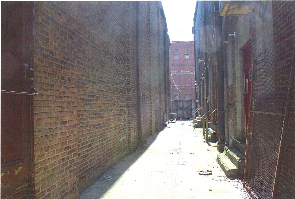
Photo 5: Alley "courtyard" between theater and main commercial block (c.d. E).
