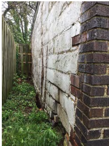
Garage north wall
