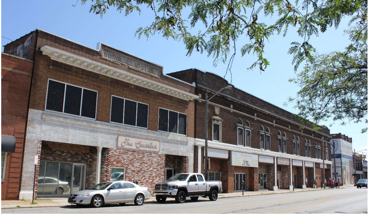
Photo 1: Homestead Block, south elevation, showing the Highland Studio Addition to the left and original block to the right (c.d. NE).
