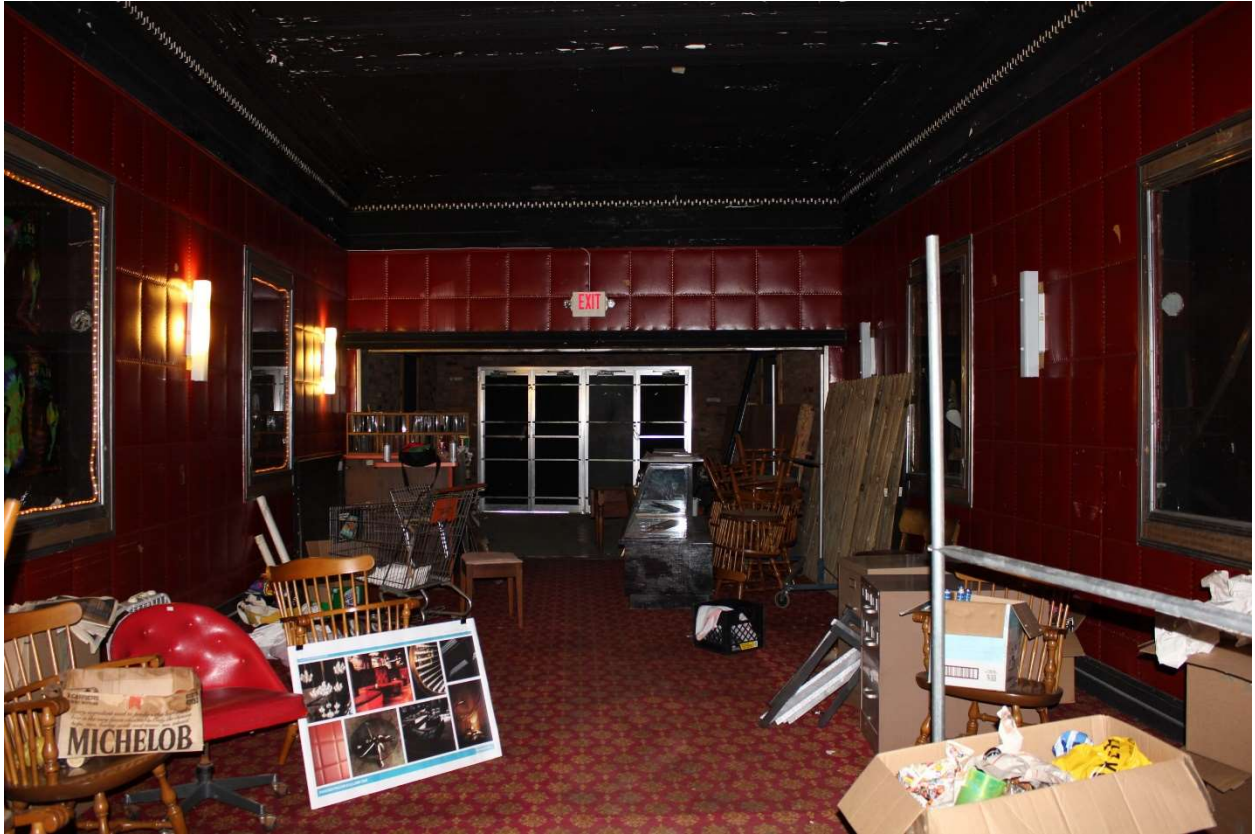
Photo 8: Homestead Theater lobby with coffered plaster ceiling, chrome poster cases and marble floor (under carpet).
