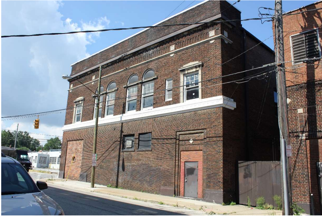
Photo 3: East elevation of main block and gated courtyard (c.d. SW).
