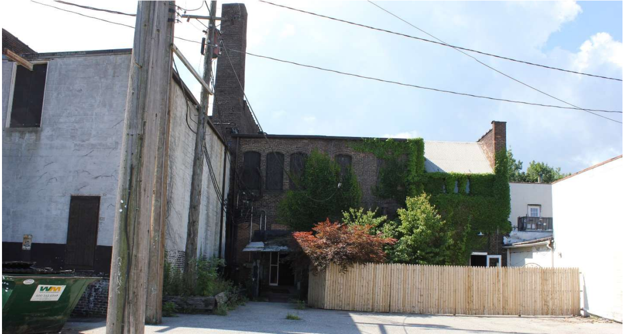
Photo 7: North elevation of Highland Studio Addition (c.d. S).
