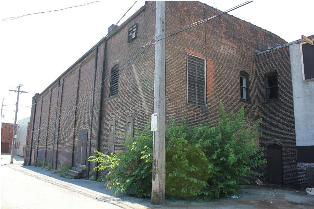
Photo 6: Northwest elevation of theater building (c.d. SE).
