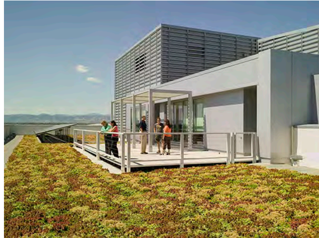
EPA Region 8 Headquarters extensive green roof – Denver, CO
