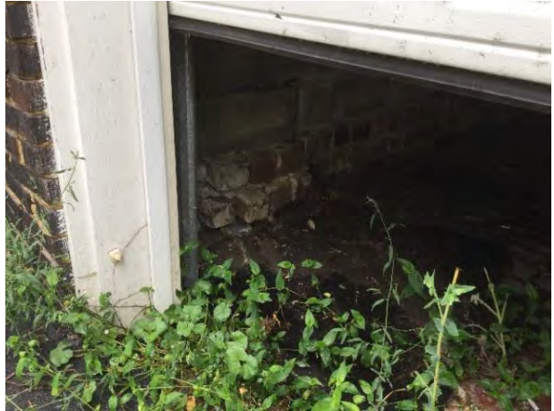
Garage northwest corner
