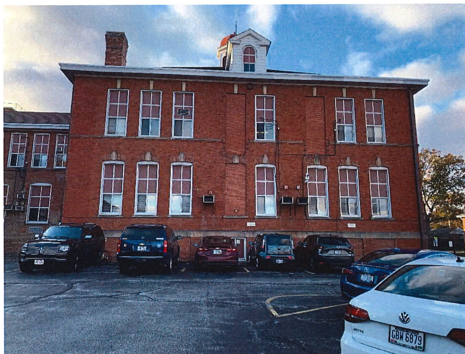
Photo 6: Grant School north elevation, 2018.
