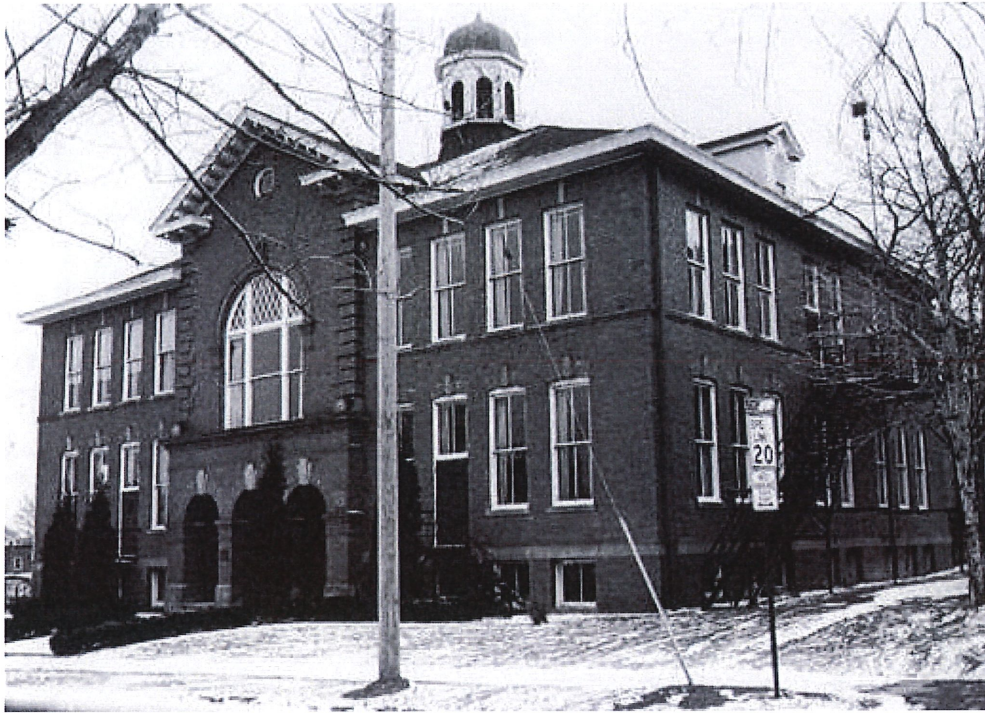
Figure 14: 1969 photo showing West elevation of Grant School addition.
