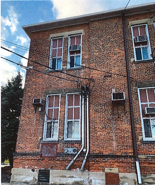
Photo 3: East Rockport Central School, north elevation, 2018.
