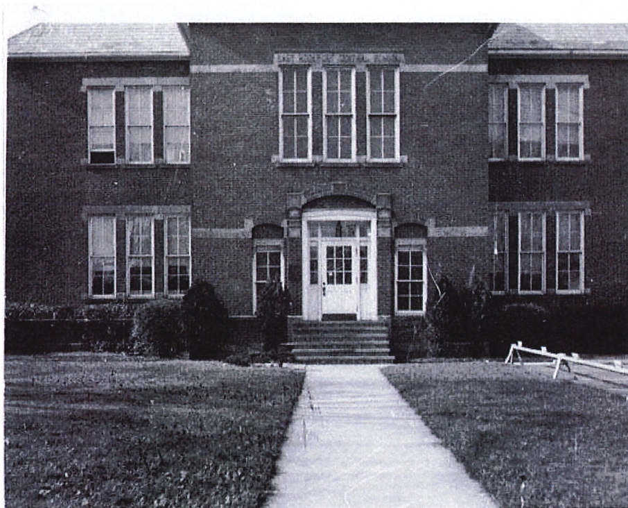
Figure 11: 1948 photo showing East elevation of East Rockport Central School.
