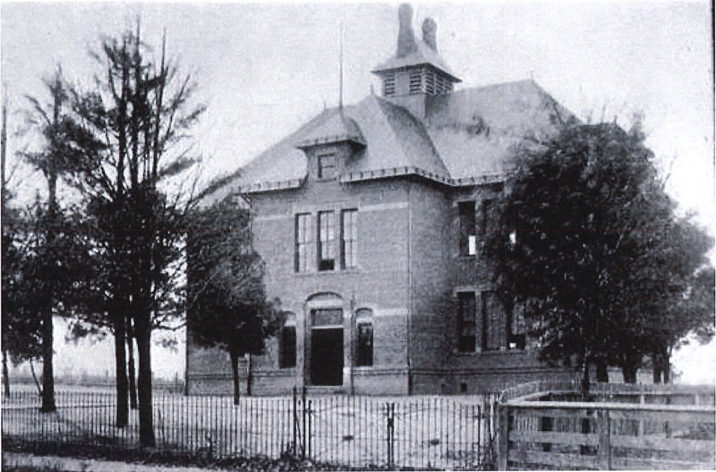
Figure 4: 1880's photo showing East elevation of East Rockport Central School.
