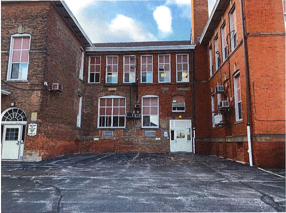
Photo 9: Grant School North elevation, 2018.
