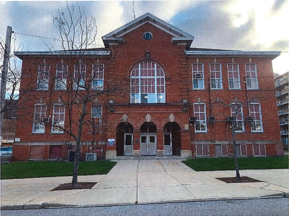
Photo 10: Grant School west elevation, 2018.
