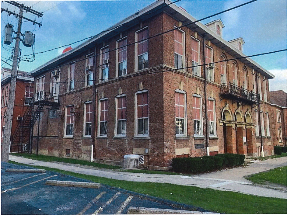
Photo 15: Grant School south and east (Warren Road) elevations, 2018.
