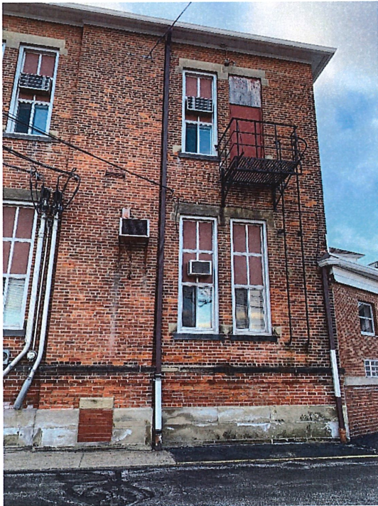
Photo 4: East Rockport Central School, north elevation, 2018.
