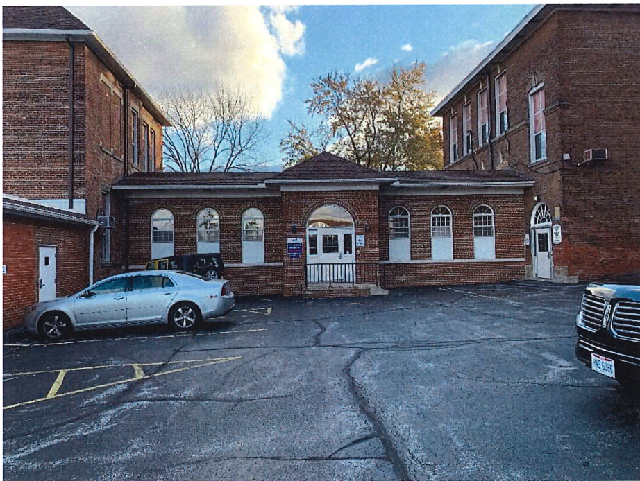
Photo 8: Connector between East Rockport Central and Grant School, west elevation, 2018.
