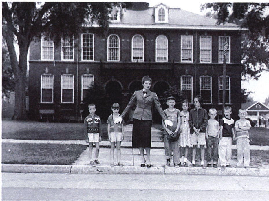
Figure 13: 1958 photo showing East elevation of Grant School.
