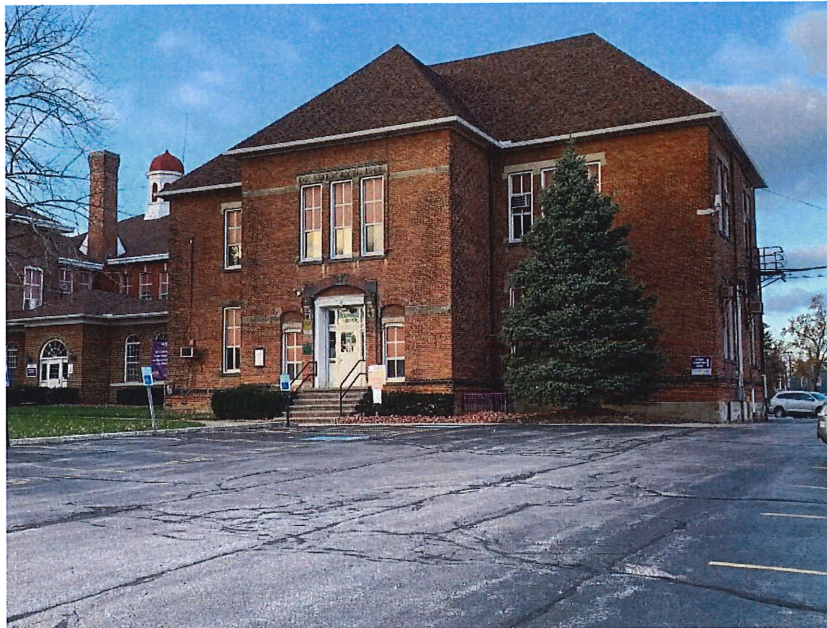
Photo 1: East Rockport Central School, east elevation, 2018.
