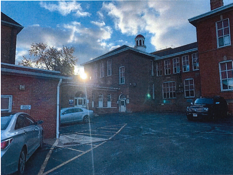
Photo 7: Grant School north elevation, 2018.
