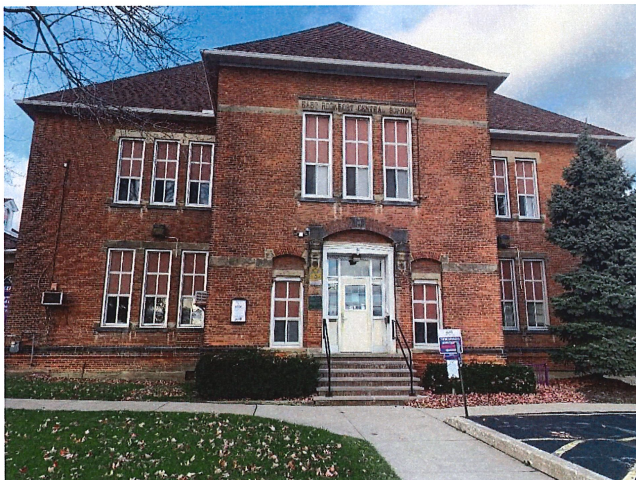
Photo 18: East Rockport Central School east elevation, 2018.
