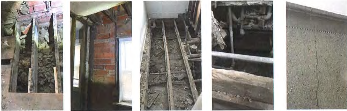
Existing Floor Structure Conditions
