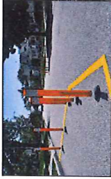
Temporary chicanes installed as a traffic calming measure on Woodward Ave. Source: Lakewood Facebook
