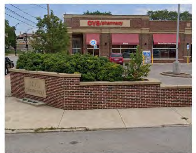
Brick wall with stone cap
