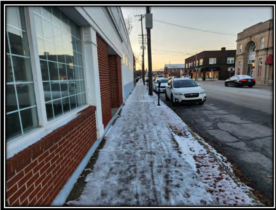
North side fronting Detroit Avenue (facing west)
