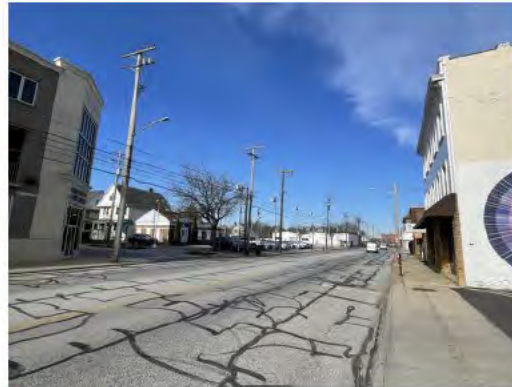
4. Rosewood Avenue & Detroit Avenue Looking West on Detroit Avenue
