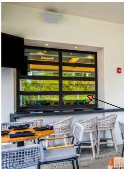
CLOPAY COMMERCIAL VERTISTACK CLEAR VETICAL STACKING WINDOW ON BUNTS ROAD FACADE.
