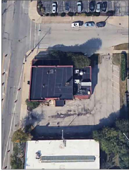
EXISTING CONDITION AERIAL PHOTO
