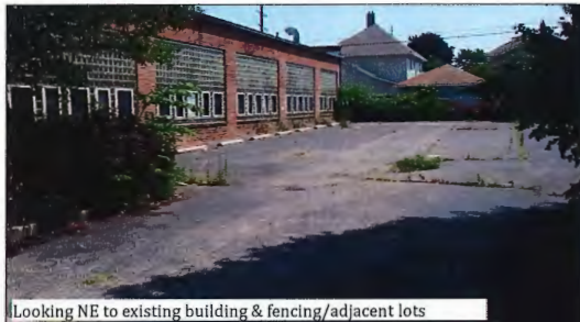
Looking NE to existing building & fencing/adjacent lots
