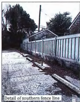
Detail of southern fence line
