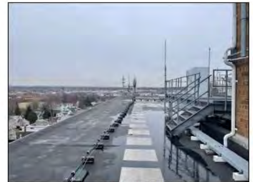
Existing Cable Run (Other Carrier)
