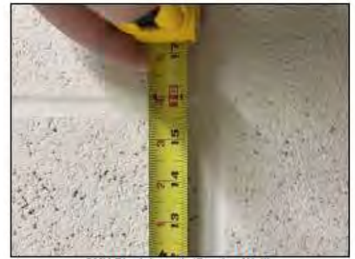
CMU Block Length (Bearing Wall)
