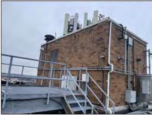
Southern Penthouse Wall
