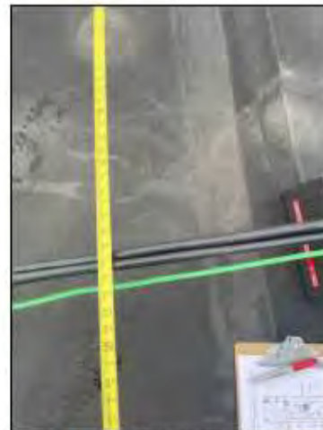
Edge Distance to Cable Run
