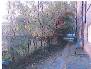
REAR OF BUILDING FACING SOUTH
