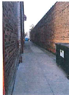
NORTH DRIVE OF BUILDING
