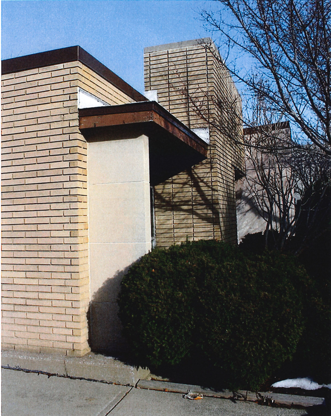
Photo 7: South elevation, detail of southwest corner, looking northeast, 2018.
