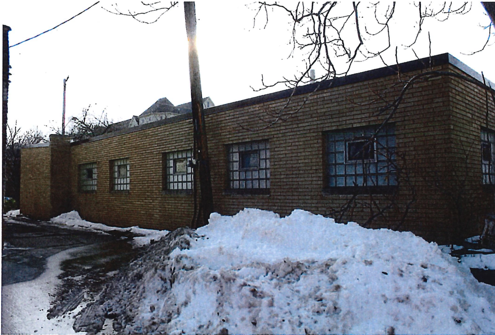
Photo 10: East elevation, looking southwest, 2018.
