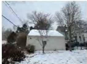
SIDE VIEW OF EXISTING GARAGE
