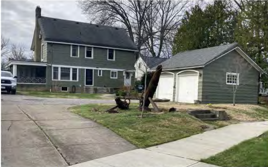
EXISTING GARAGE AND WALKWAY STEPS VIEWED FROM EDGEWATER DRIVE
