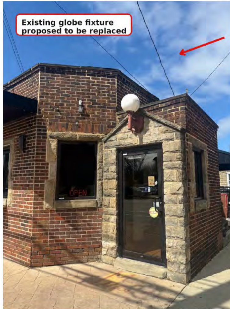
Figure 1. Existing corner condition and fixture to be replaced.
