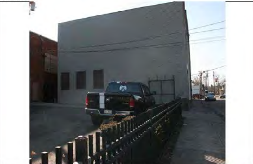
Photograph 4 – View of rear of property, looking south.
