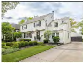
FRONT VIEW OF HOUSE & GARAGE
