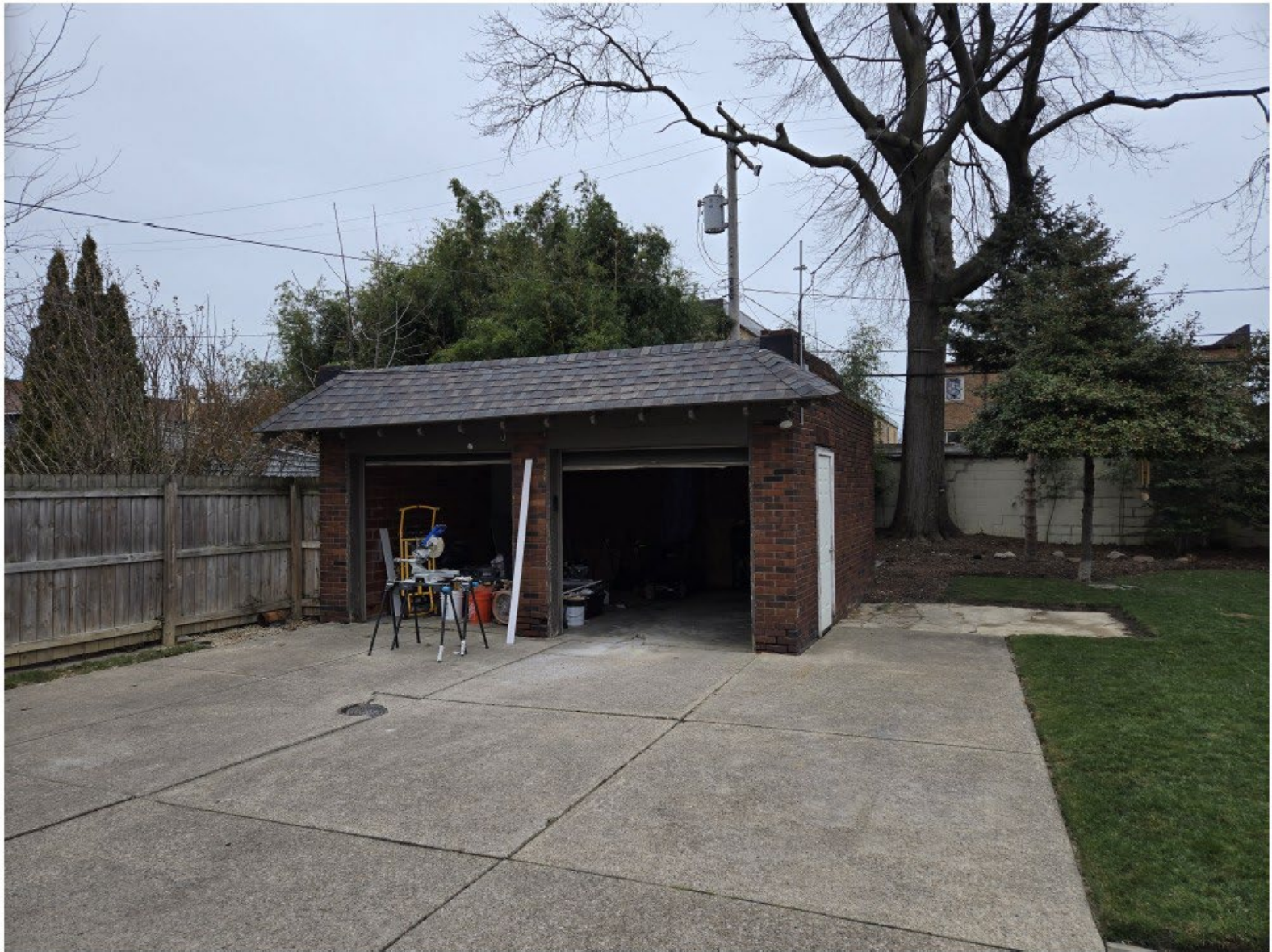
EXISTING CONDITIONS PHOTOGRAPH VIEWING NORTH N.T.S.
