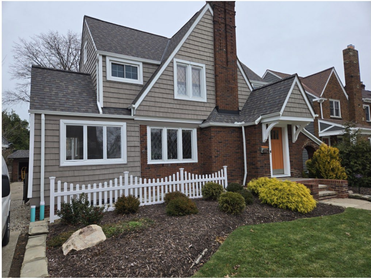
EXISTING CONDITIONS PHOTOGRAPH VIEWING NORTH N.T.S.
