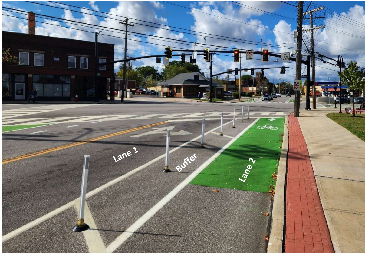
Figure 6 – Hilliard Rd Southwest Approach
