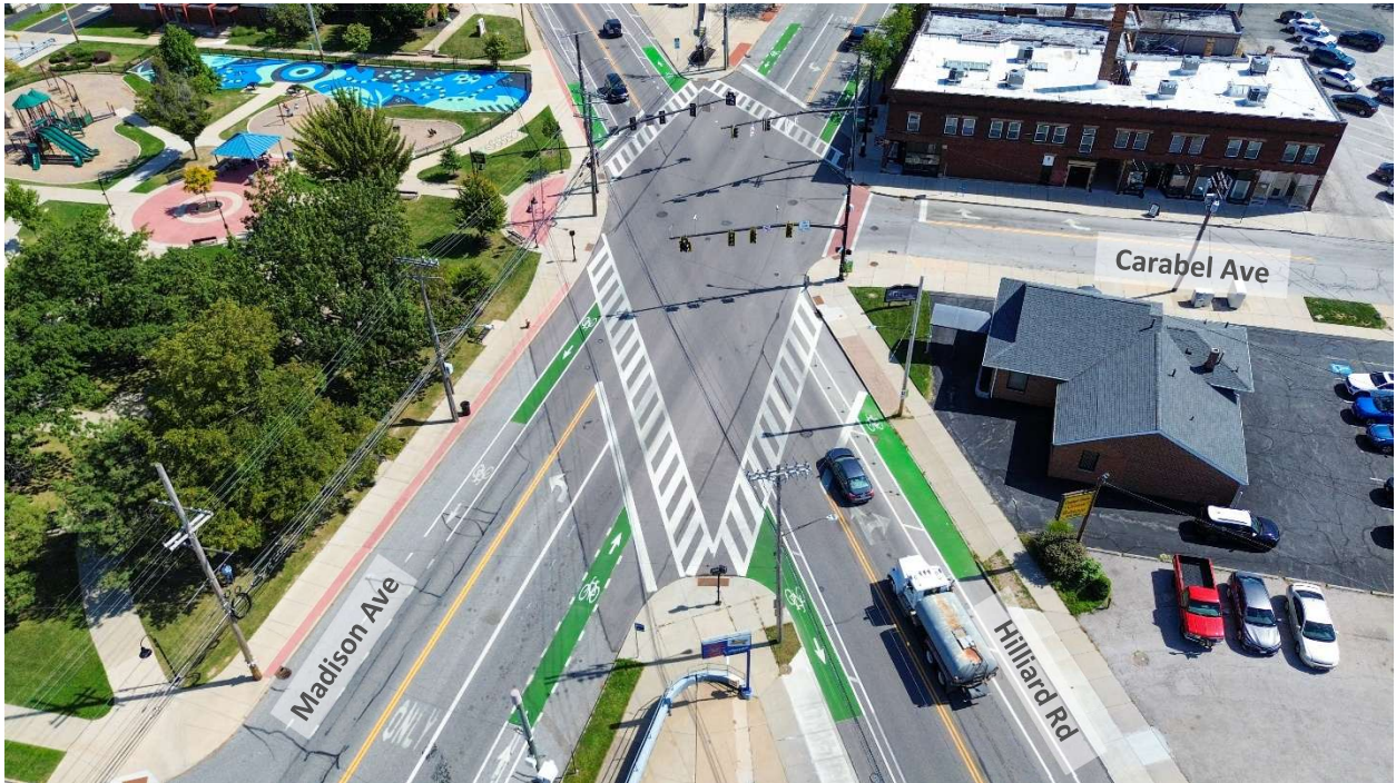
Figure 2 – Madison Ave & Hilliard Rd/Carabel Ave Aerial View
