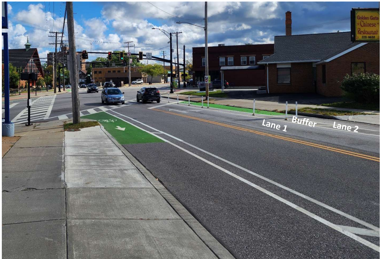
Figure 5 – Hilliard Rd Northeast Approach
