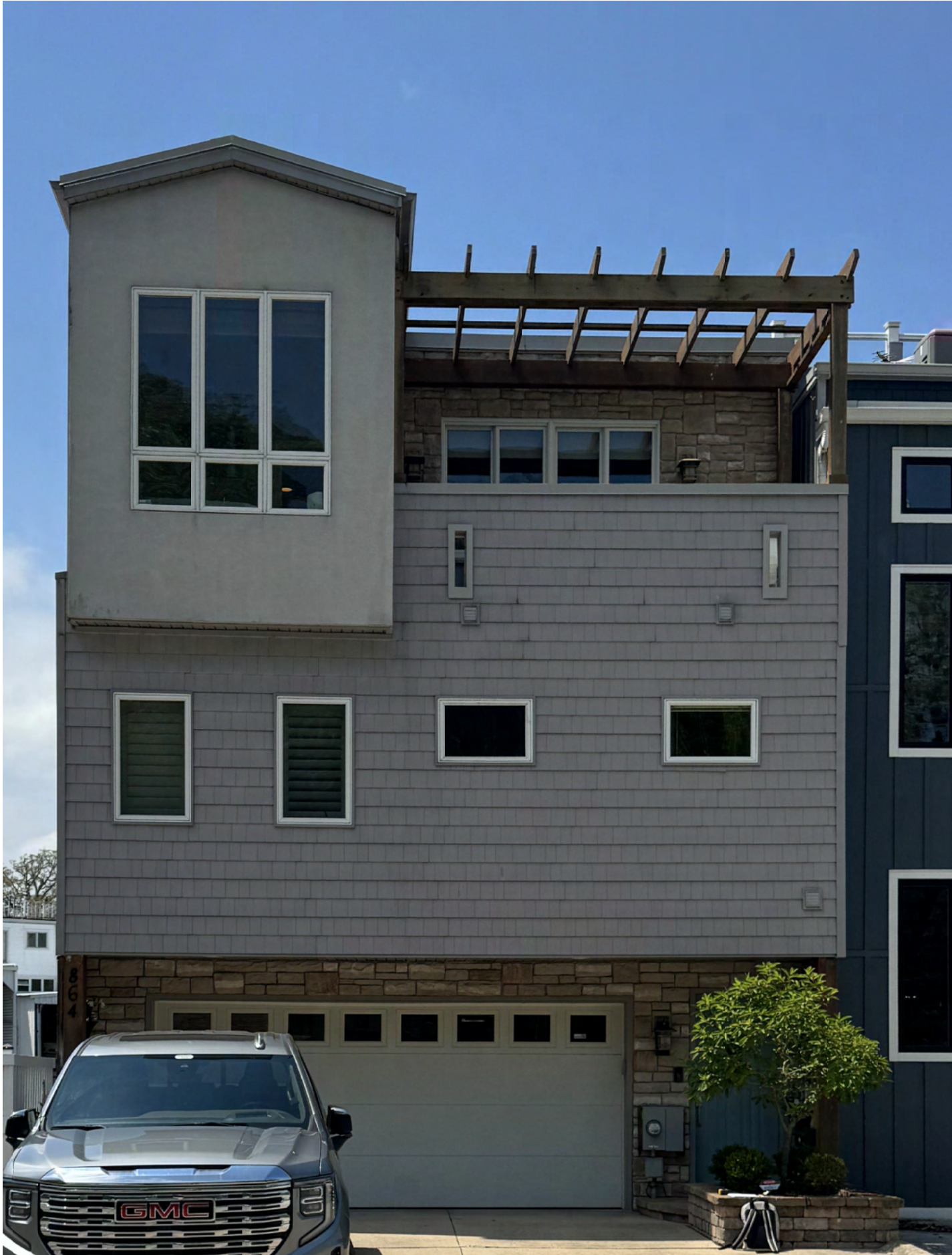
East Elevation - Photo Existing Conditions NTS
