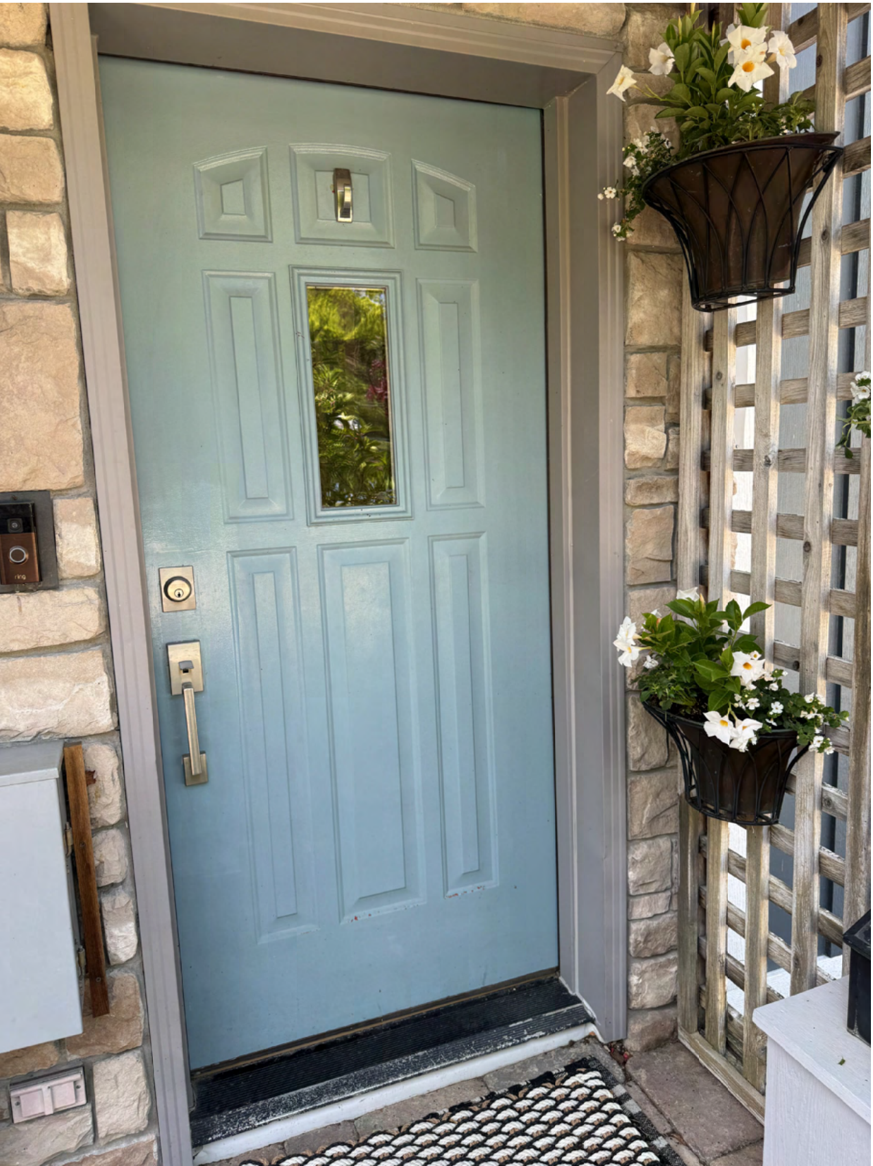
View of existing front entrance door
