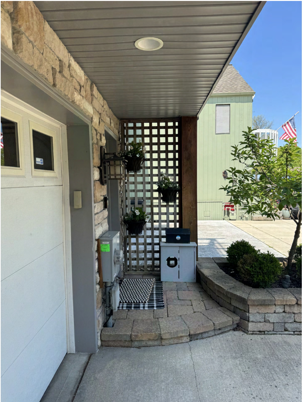
View of front entrance stoop
