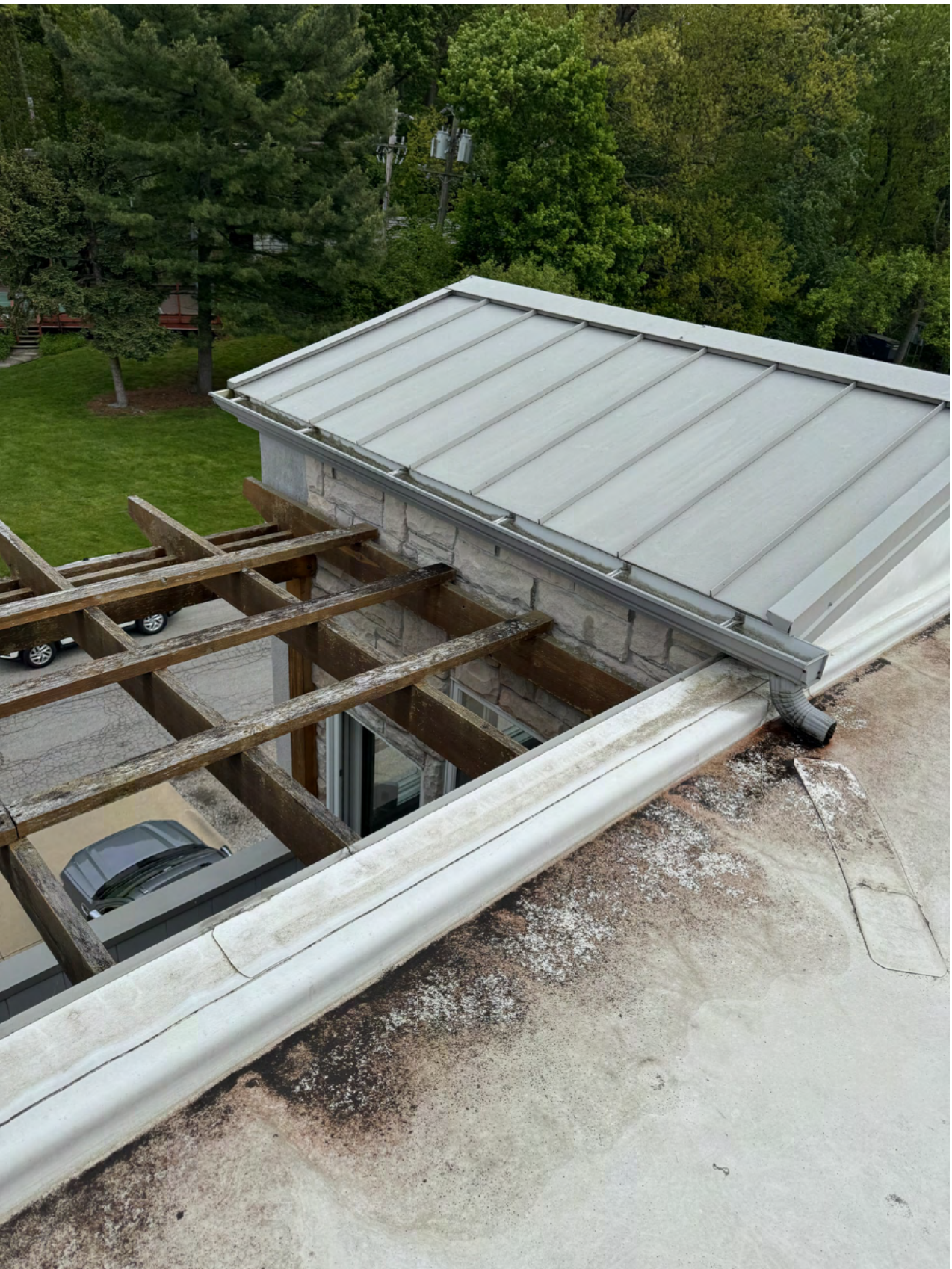
View of existing roof / trellis at front
