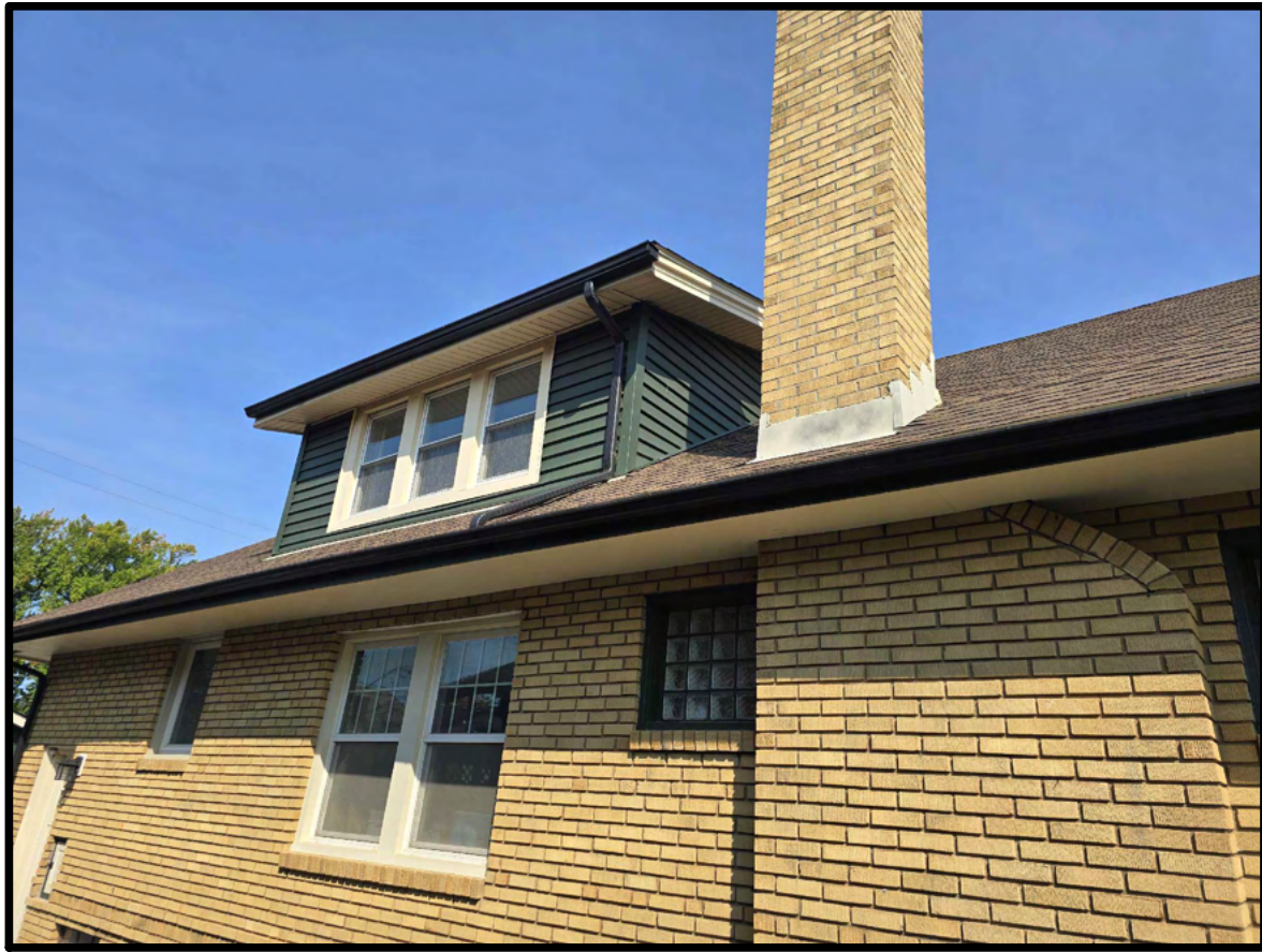
EXISTING SOUTH DORMER
