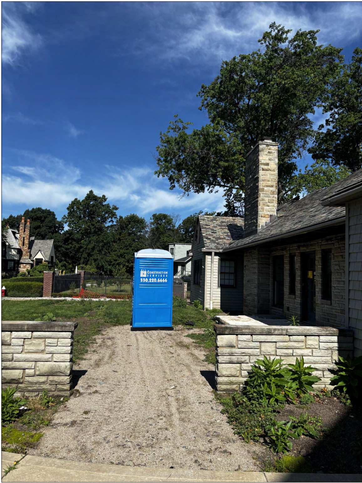
EXISTING HOUSE APPROACH TO FRONT DOOR LOOKING NORTHWEST
