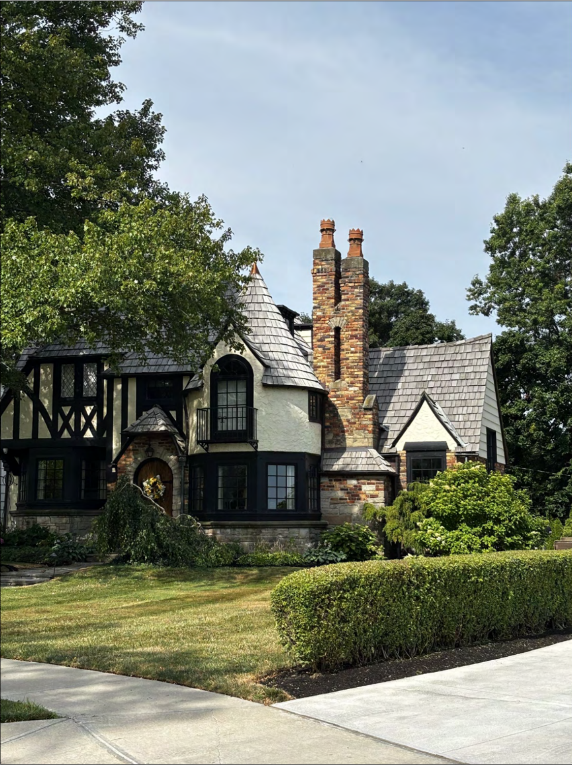
NEIGHBORS HOUSE TO THE SOUTHWEST
