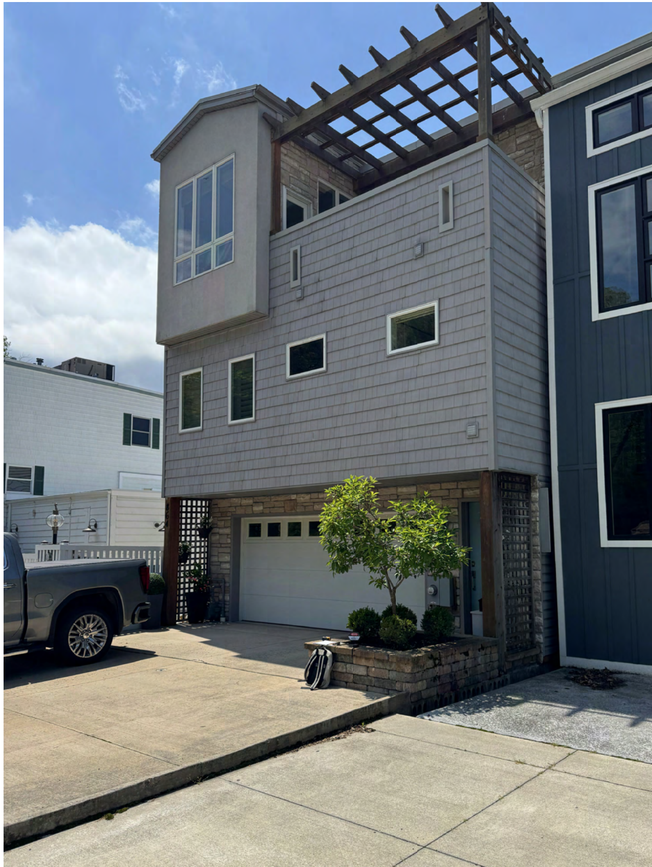
View of front, from the NE
