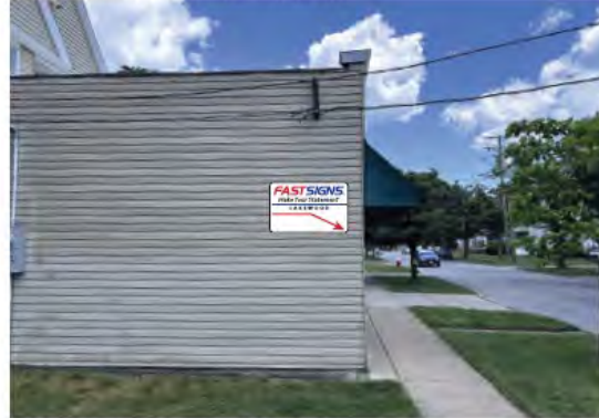
SOUTH FACADE (FACING MADISON)
