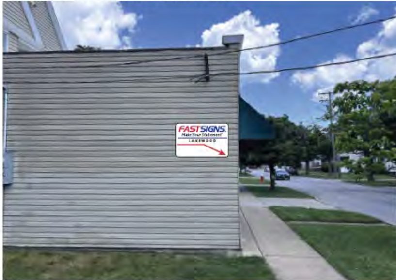
SOUTH FACADE (FACING MADISON)
