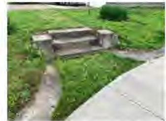
EXISTING REAR STEPS
