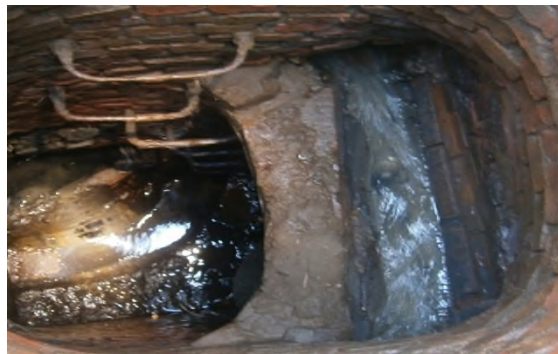
Figure 2.11: Side Flow Weir - Shelf
