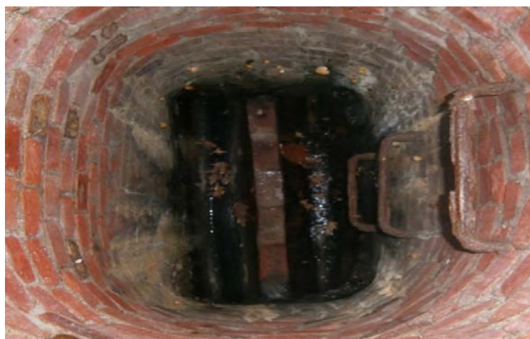
Figure 2.12: Side Flow Weir - Invert
