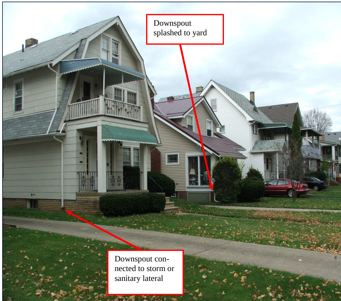
Figure 7-5: Typical Downspout Configurations
