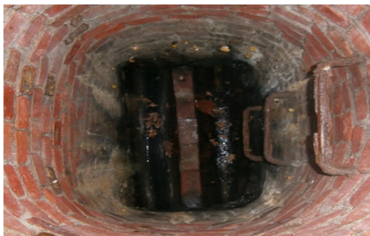
Figure 2.12: Side Flow Weir - Invert
