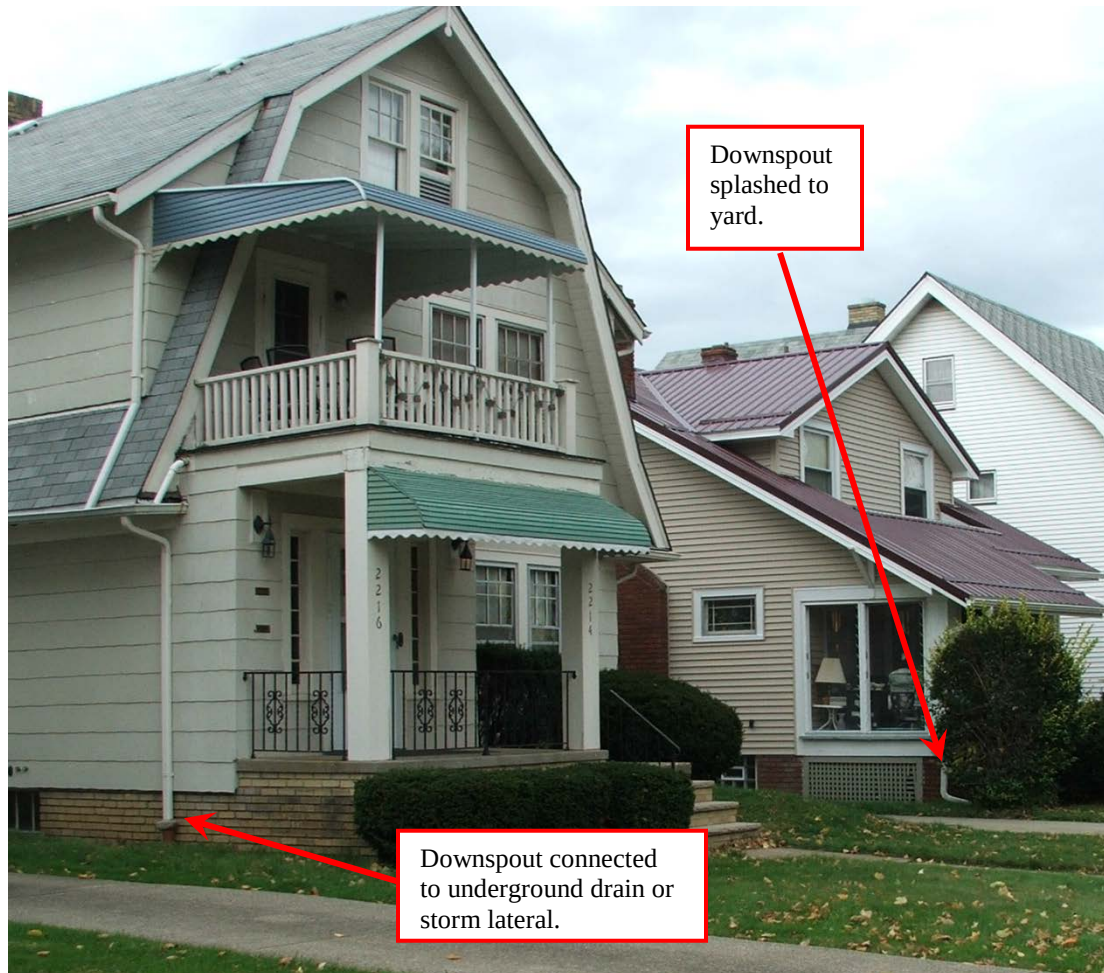
Figure 4-4 Typical Downspout Configurations
