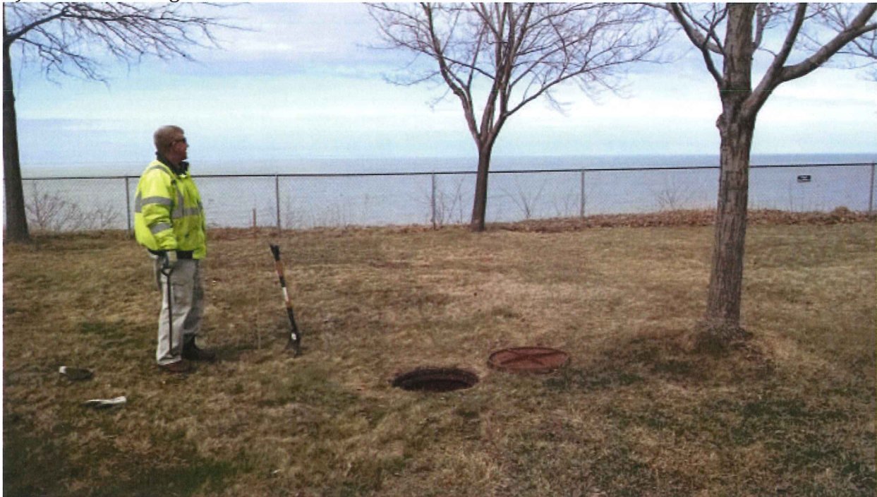
1) Site View facing north:
