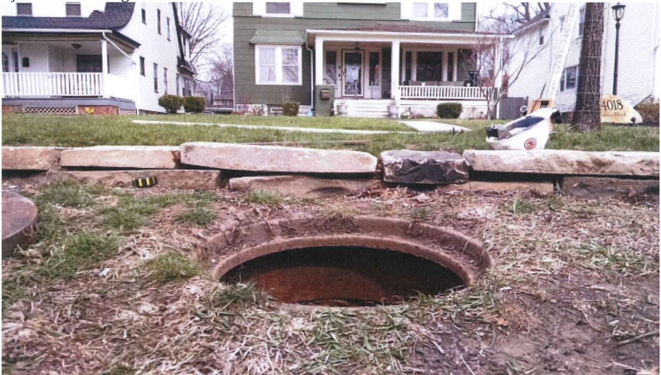
1) Site View facing north:
