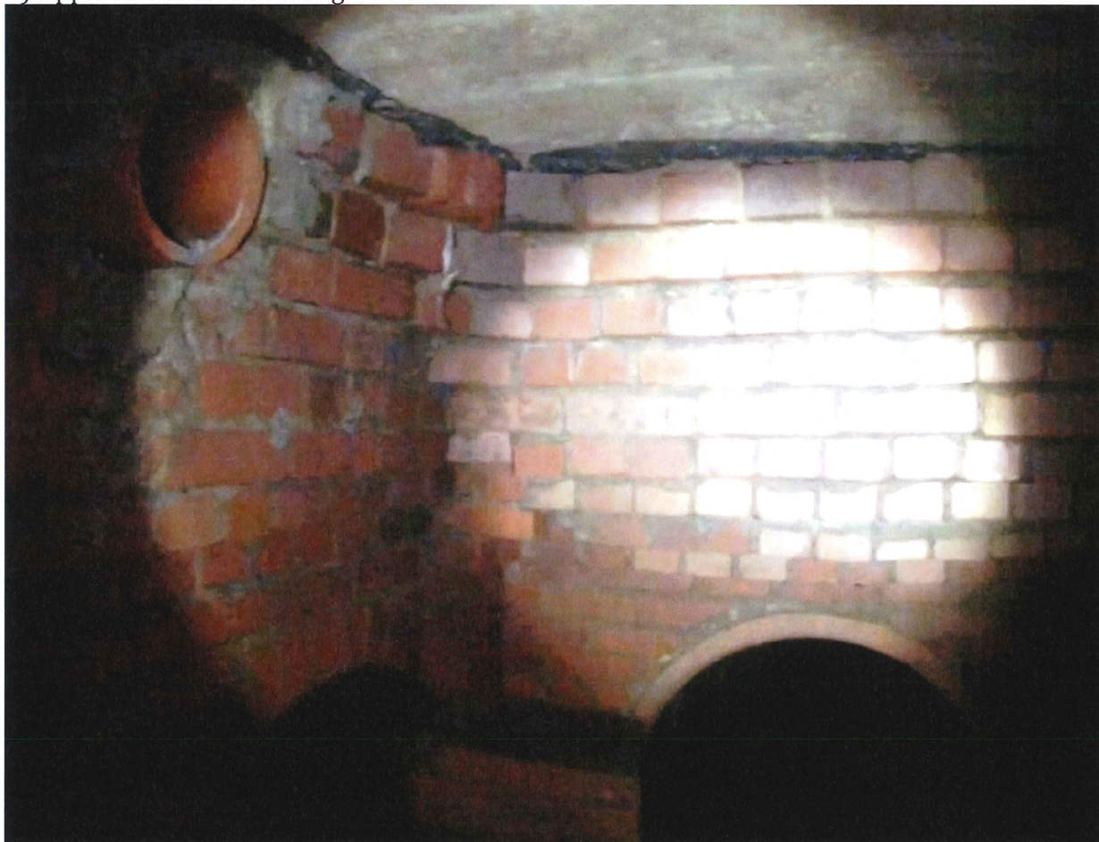
6) Upper MH Chamber facing SE – Shows eastern and southern 30" inlets and 6" eastern inlets.
