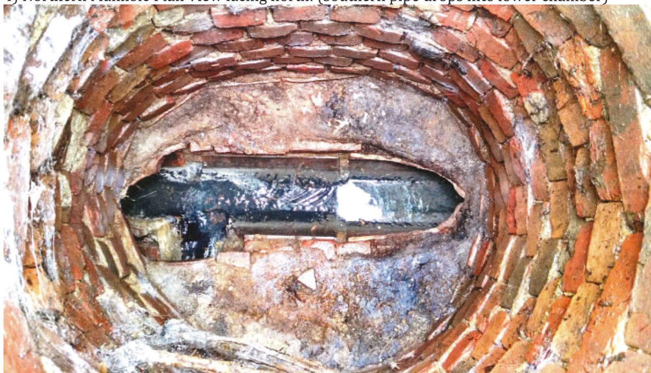
4) Northern Manhole Plan View facing north: (southern pipe drops into lower chamber)
