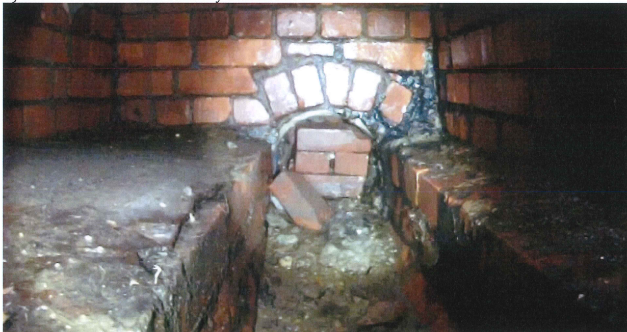
5) Lower MH – Eastern Sanitary bulkheaded:
