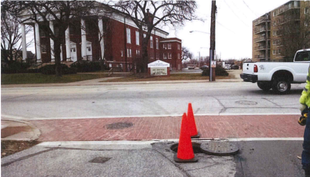
1) Site View facing north:
