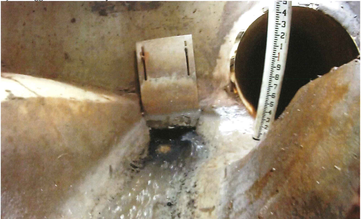
4) Unclogged NNW sanitary outlet:
