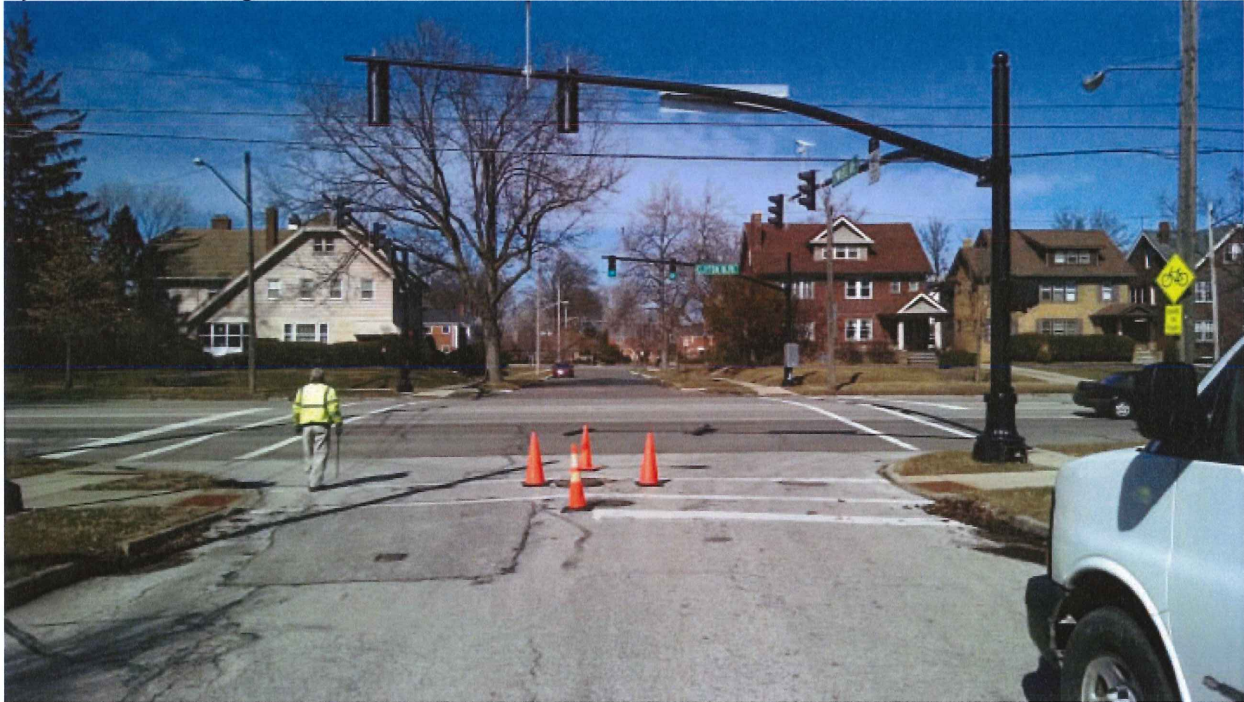
1) Site View facing north:
