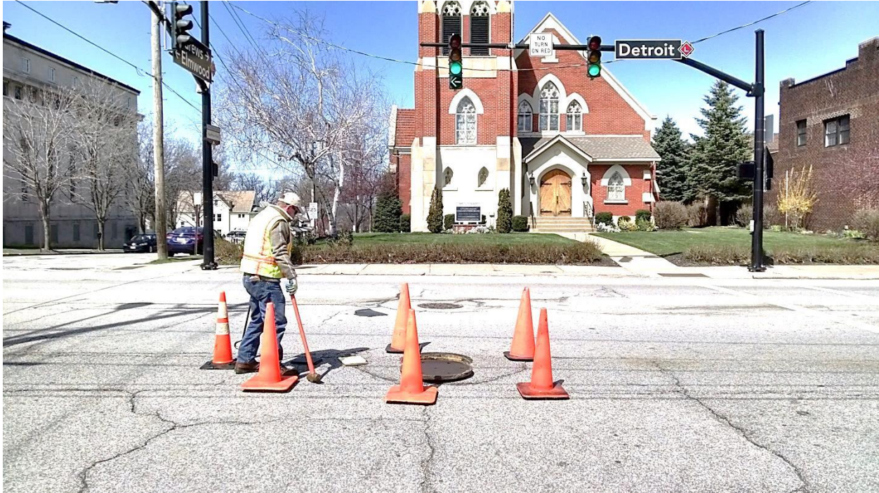
1) Site View facing north:
