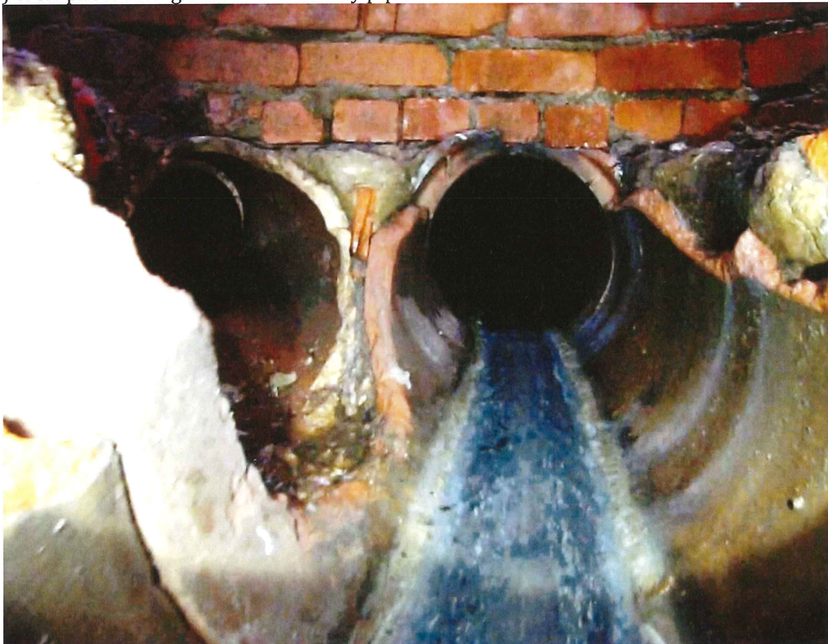
4) Weir photo facing west from sanitary pipe:
