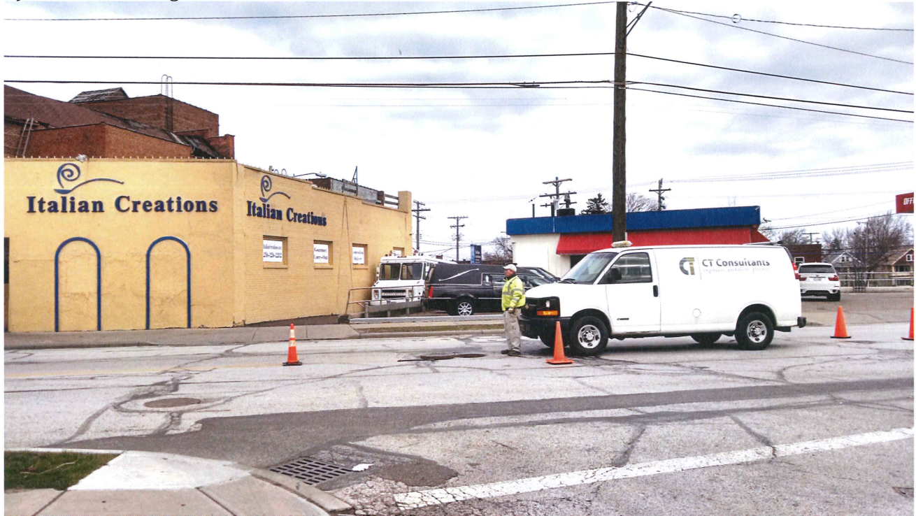
1) Site View facing north:
