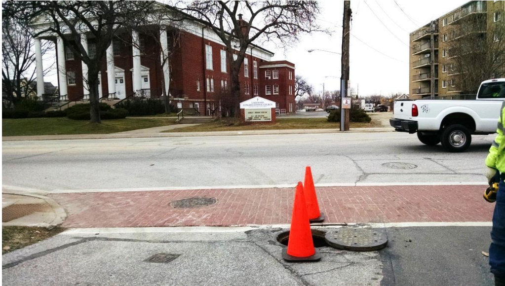
1) Site View facing north:
