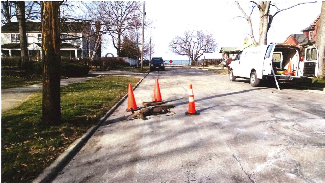
2) Site View facing north:
