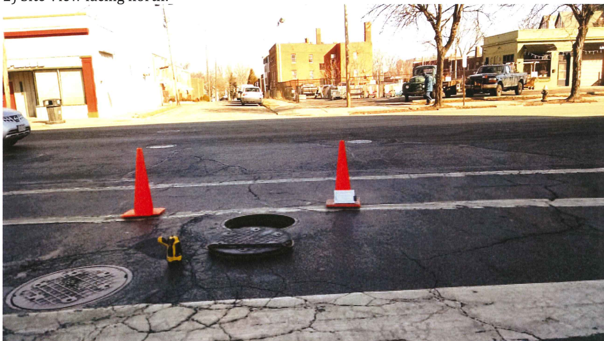
2) Site View facing north:
