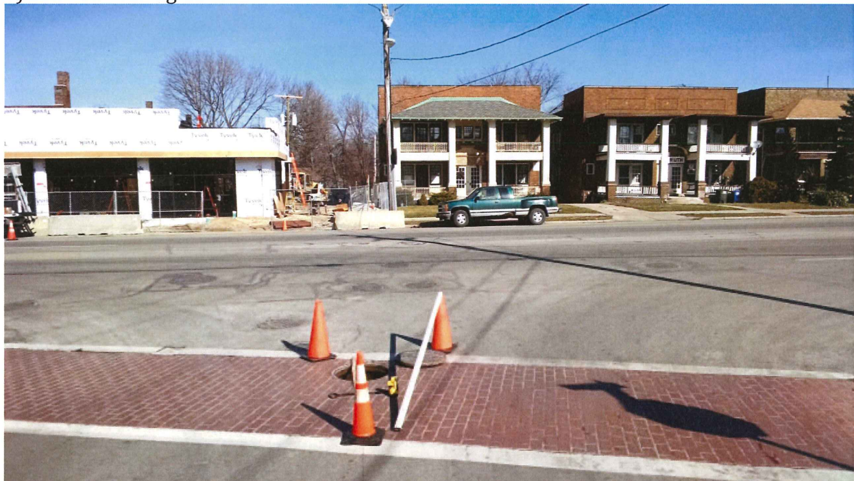
2) Site View facing north:
