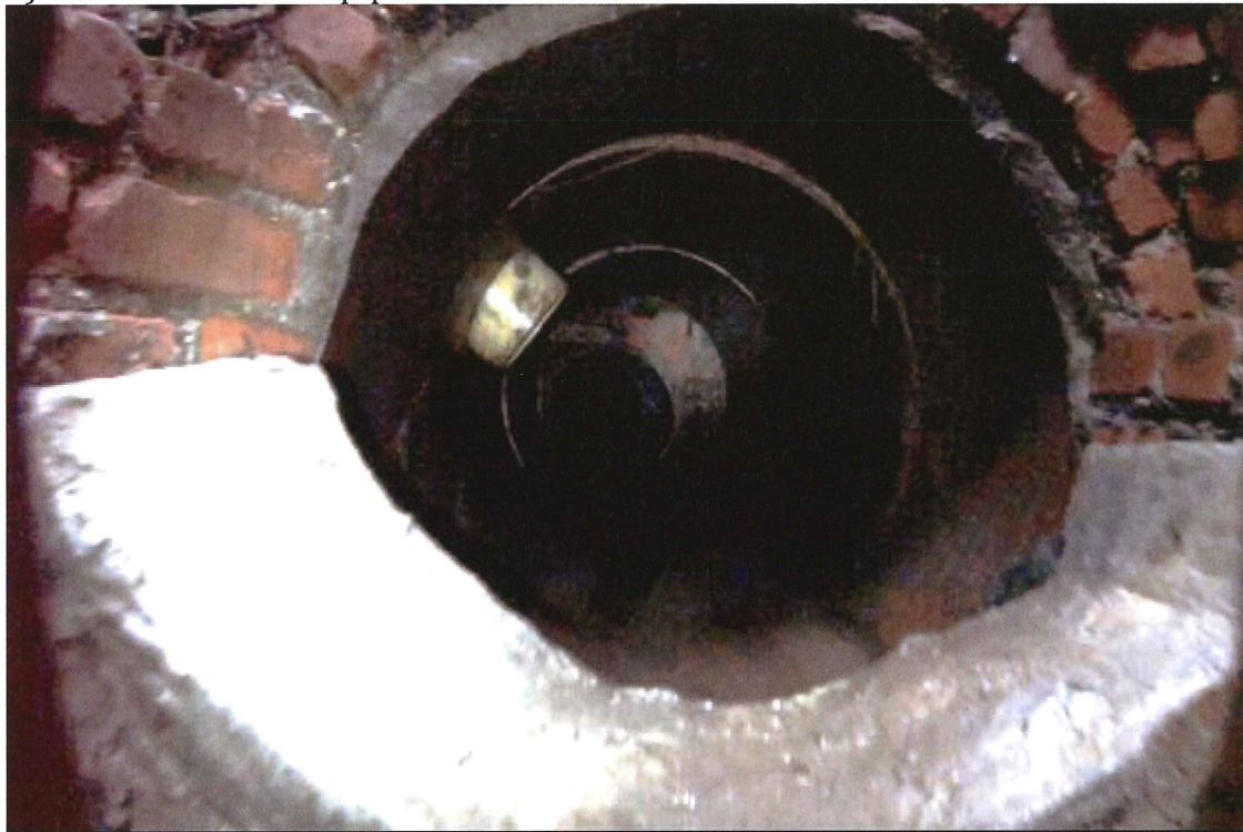
4) Northern Overflow pipe:
