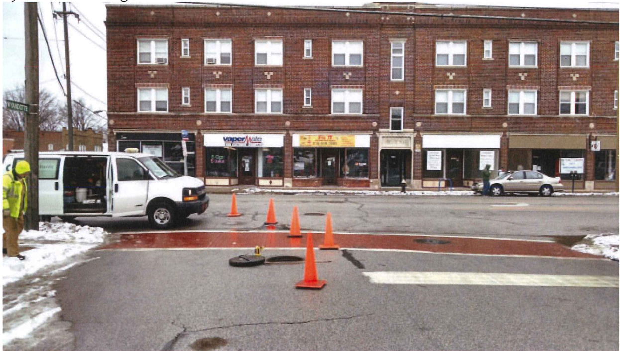
1) Site View facing north:
