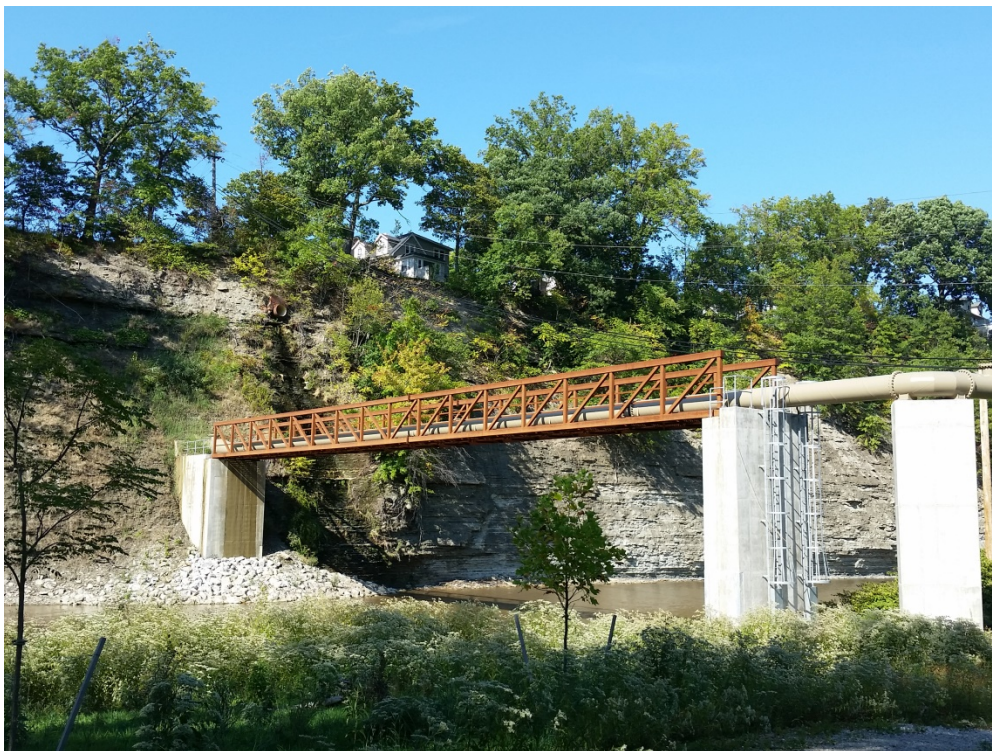
FIGURE 2-8. West End aerial sewer
