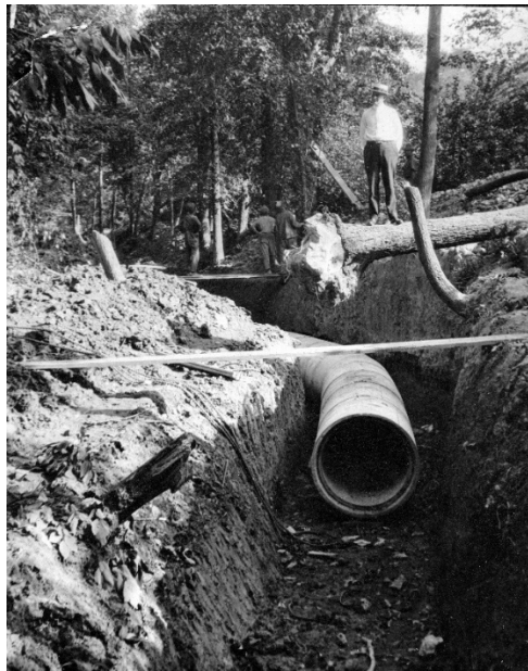
FIGURE 2-4. Lakewood’s interceptor under construction near the WWTP
