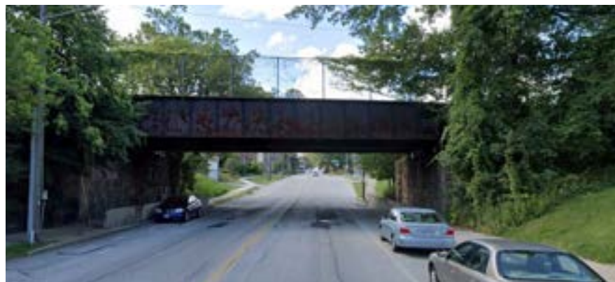
Railway overpass on West Clifton Boulevard. Source: google maps
