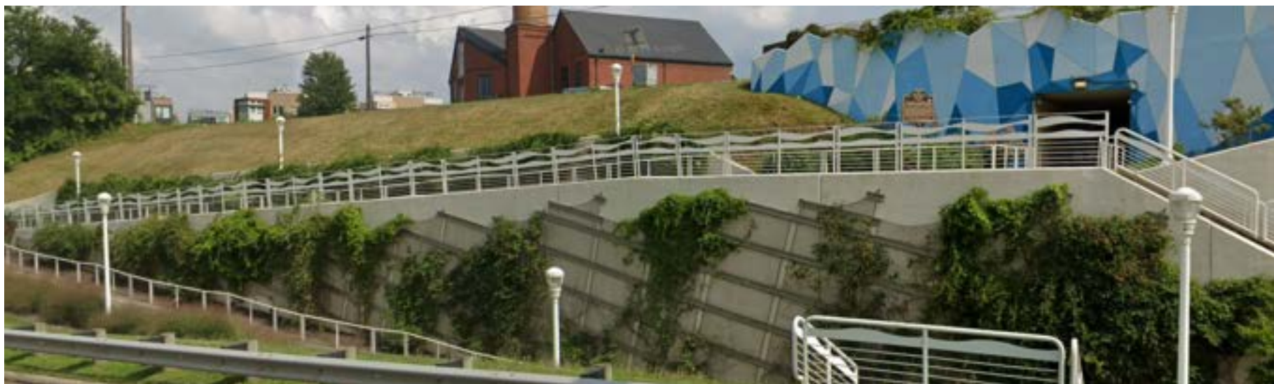
Cleveland Metroparks installed a living wall to help clean the air and beautify the pedestrian tunnel and ramp connecting Edgewater Park to neighborhoods to the South. Source: Google Maps
